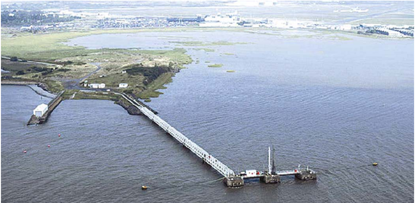
Shannon Airport Oil Jetty
