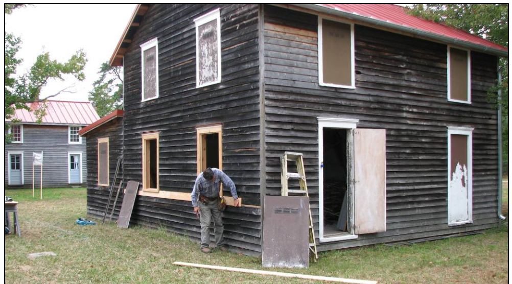
Al Morrison reconstructs window frames on worker cottages undergoing restoration.
