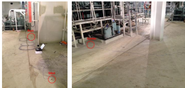
Figure 4: Onboard structure-borne noise measurement in the steering gear room
