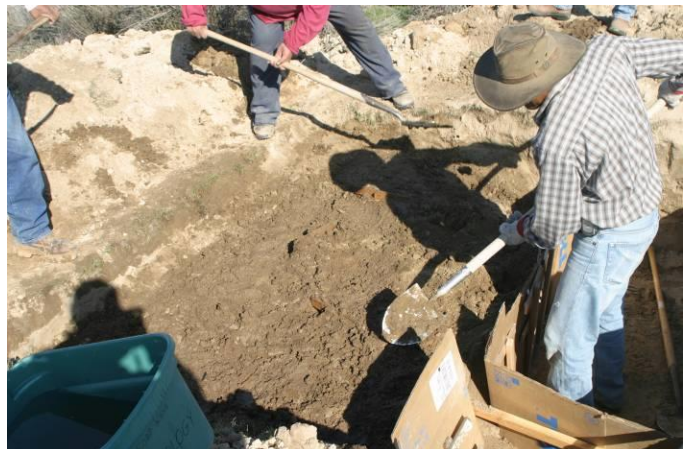
Photo 16. After the step in photo 5, put about 2.5 inches of fine sand on the top of cuttings.
