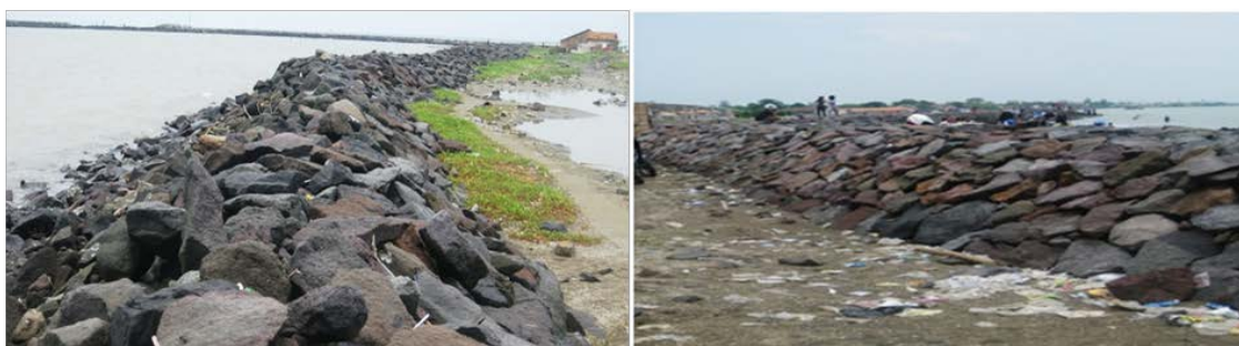
Figure 12. Dozen km of high cost sea wall for protecting the beach in Indramayu District.
