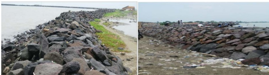
Figure 12. Dozen km of high cost sea wall for protecting the beach in Indramayu District.
