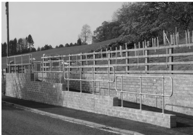
The wall opposite Portmoak Hall, with new handrails in place
