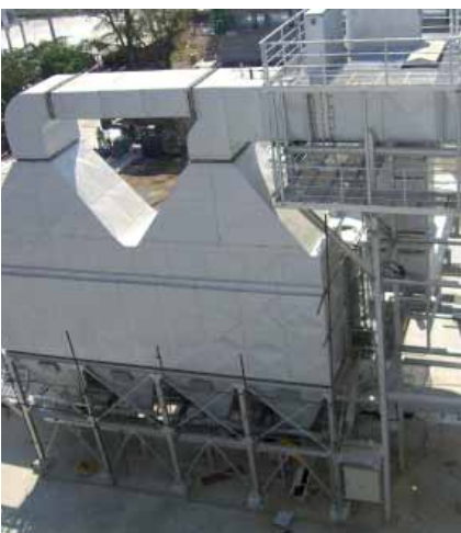
Centrale elettrica di Bua Yai, Tailandia Flu gas cleaning, Biomass Power Plant Extraction from boiler ash dust, Fuel rice husk, Biomass
