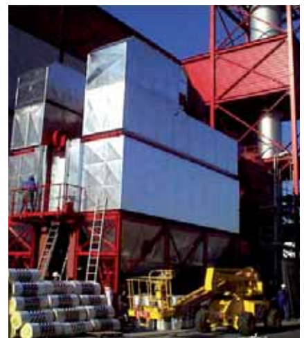
Themoselect S.A., Locarno (Svizzera) Waste gas cleaning for garbage disposal plant separating of dust and sulphur dioxide
