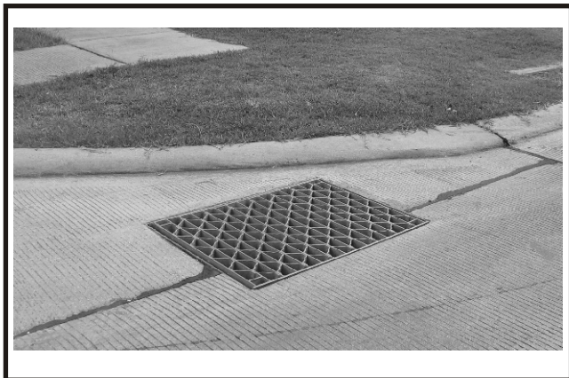
Underground Drainage Inlet
