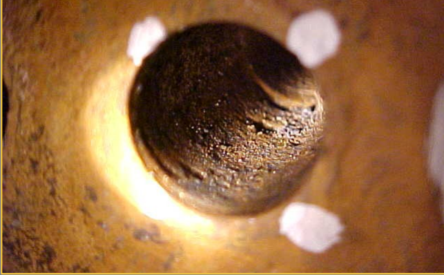
Ammonia bisulfide corrosion/pitting within roll area
