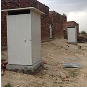
Affordable household toilets near Jaipur, Rajasthan
