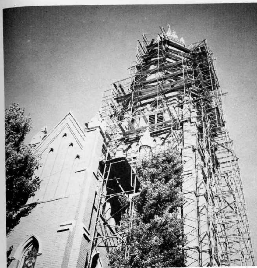
REPAIRING THE STEEPLE DAMAGED BY WINDSTORM
