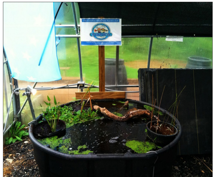
The first stage of work on the Corcoran Aquatics Lab, with the tanks, plants, and aeration system in place and shelving, benches and workstations to follow.
