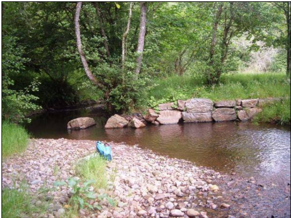
Plate 4 Rock utilised to prevent erosion.
