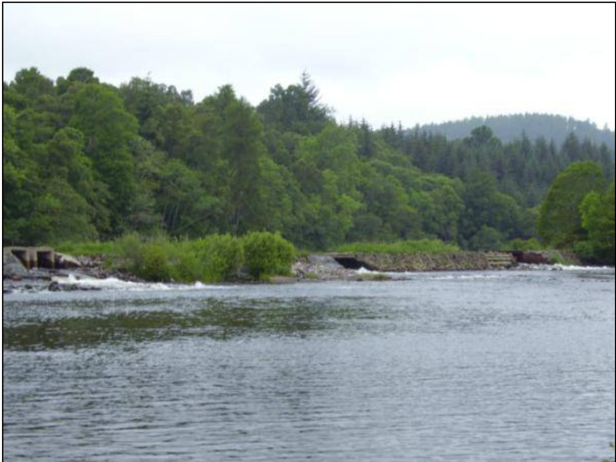
Plate 2 Looking upstream to the Cruives.
