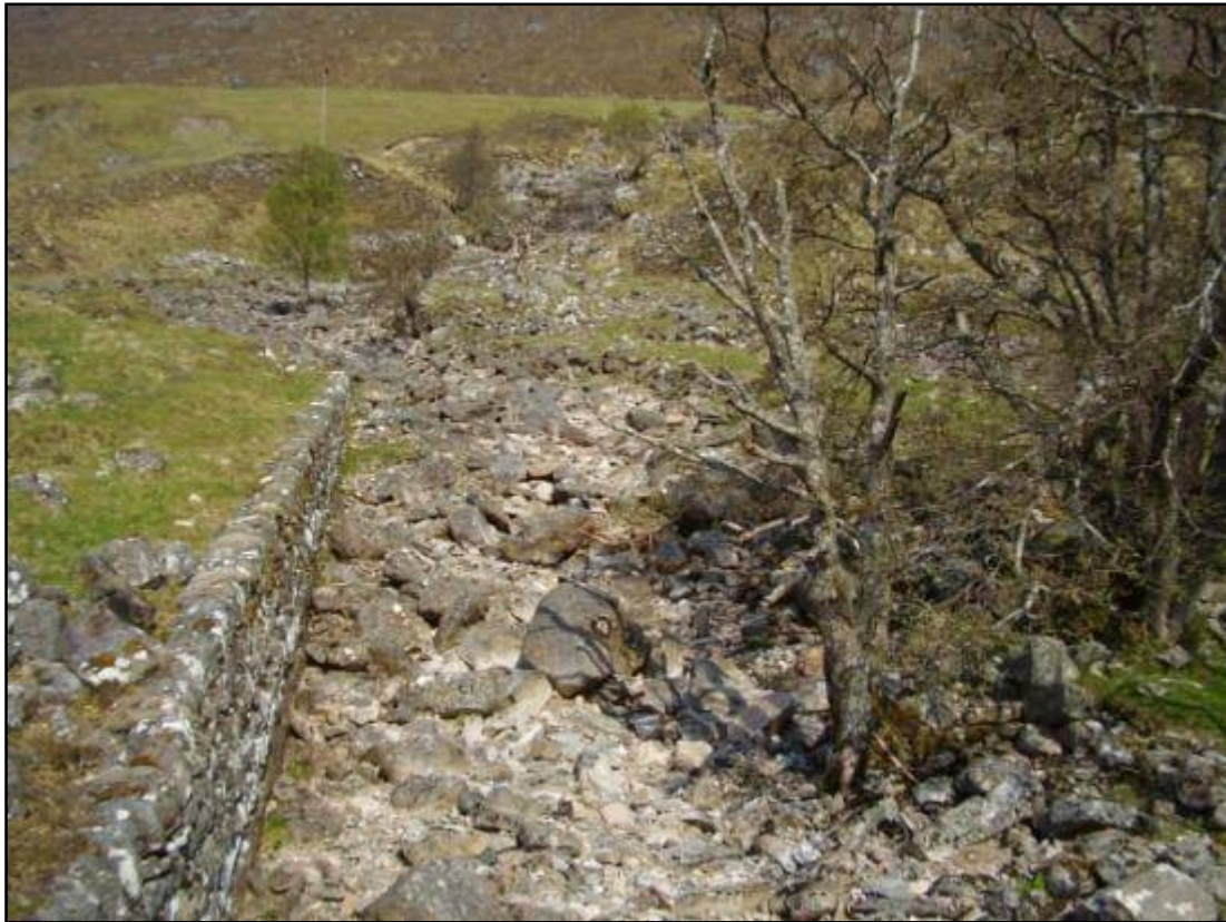
Plate 31 Toll a' Mhuic looking upstream from the road bridge
