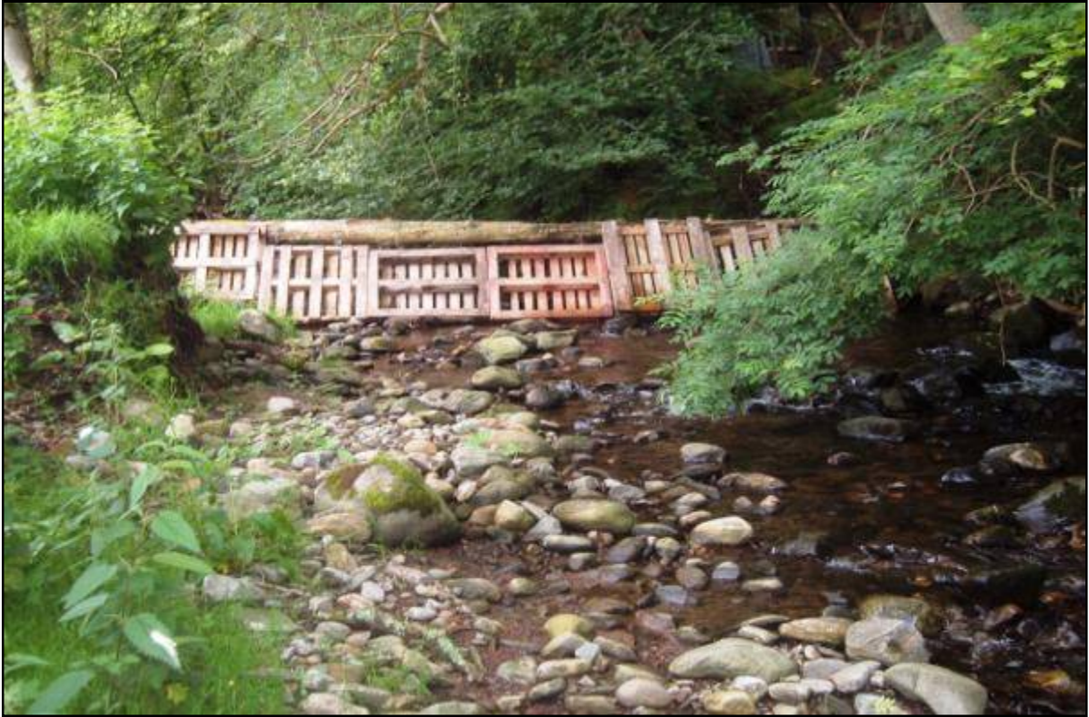
Plate 7 Water gate on Bruiach Burn.
