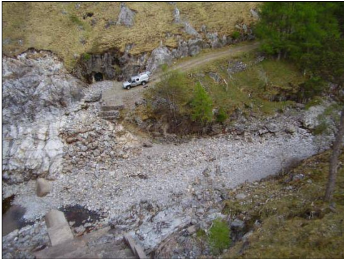
Plate 35 Looking downstream from Monar Dam (Garbh-uige).
