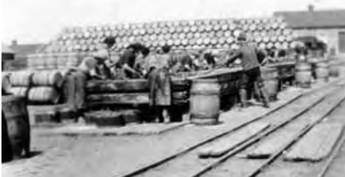
Gutters and coopers at work. Accommodation hut is in the background
