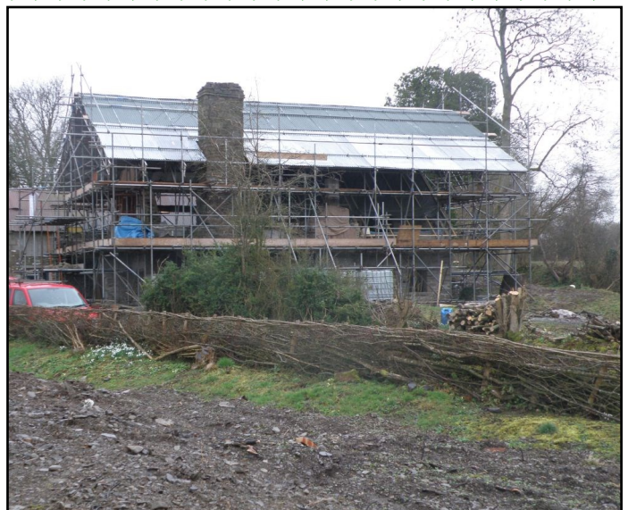
Rhosgoch Mill encased in scaffolding
