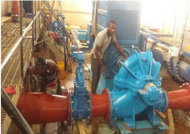
Kano High lift pumps Chalawa (Being installed)
