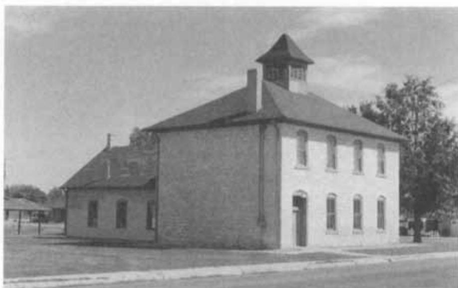
This building in Redmond was used as a school until 1911 and a church until 1917. The original one-story adobe building was constructed in 1881 and the two story rock structure added to the front in the 1890s. (Allan Kent Powell)
