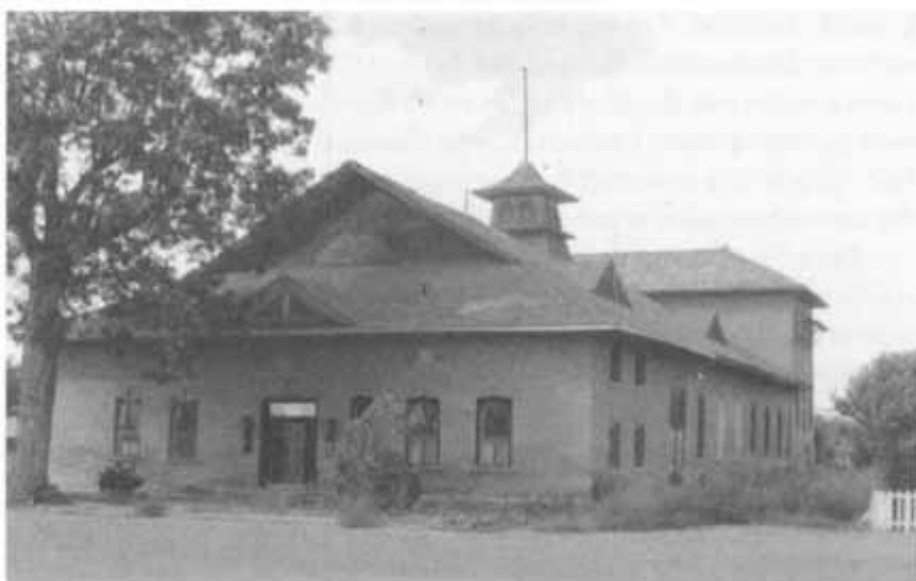
The Monroe Pavilion, built in 1907, was the recreational center for southern Sevier County for many years. (Allan Kent Powell)
