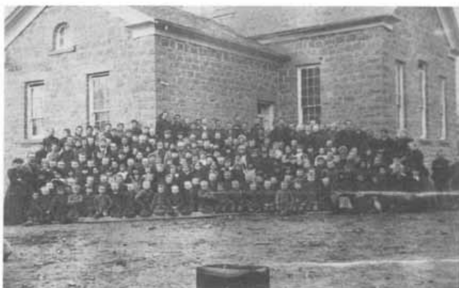
The Richfield rock school, constructed during the winter of 1864–65, serves as the backdrop for this photograph of Sevier County students. (Utah State Historical Society)
