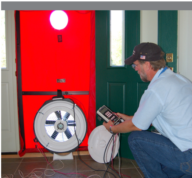
Professional energy auditors perform "blower door tests" to determine a homes airtightness. Reducing drafts increases building energy efficiency.
