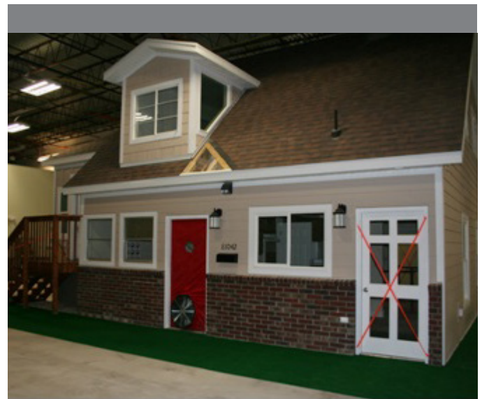
The Utah Intermountain Weatherization Training Center created a two-story 1200 foot replica of a home used to demonstrate best practices for weatherization and efficiency, providing important education to Utah community members and builders.
