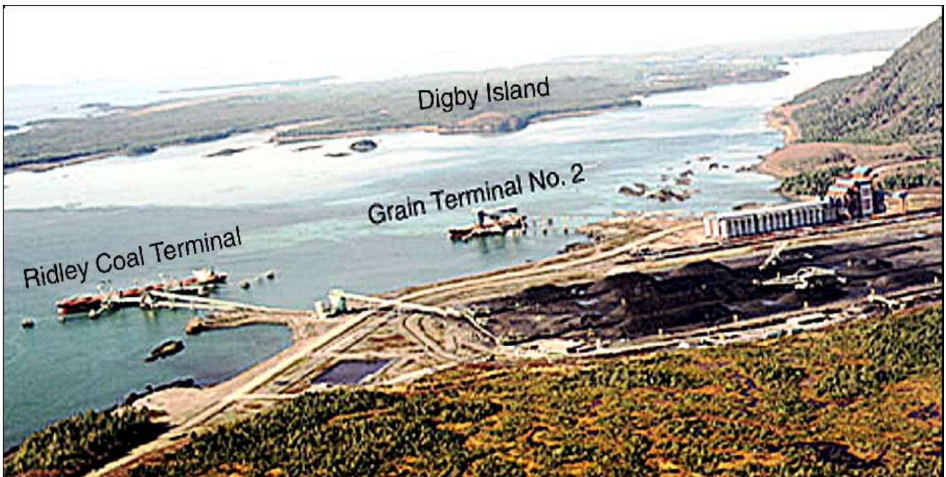
Prince Rupert Port—Ridley Island Terminal
