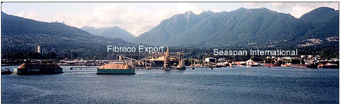
Fibreco Terminal and Seaspan Terminal
