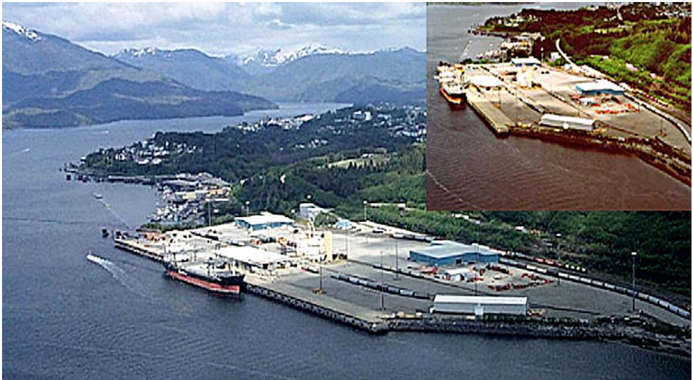
Prince Rupert Port—Fairview Terminal
