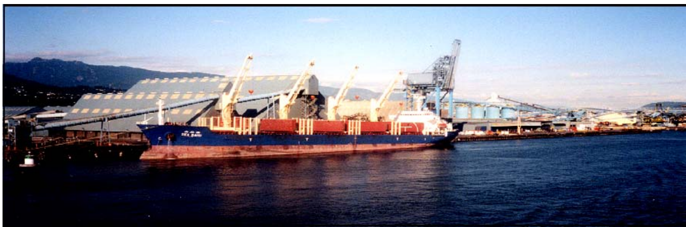
Vancouver Wharves—West Dock
