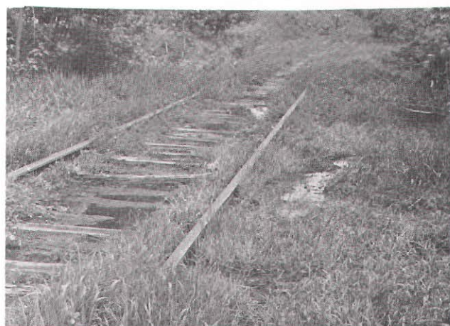
DRAINAGE CONDITIONS ALONG RAILWAY LINE WAUKESHA TO MILTON JUNCTION
