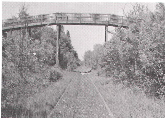
TYPICAL TRACK CONDITION— WAUKESHA TO MILTON JUNCTION
