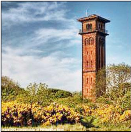
Cleadow Hill Water Tower
