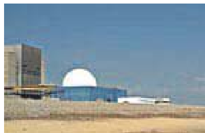
Sizewell Nuclear Power Station
