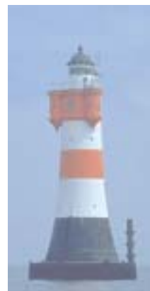
Roter Sand Tower
