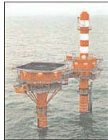
Oostdyck Radar Tower
