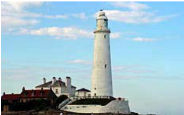
St. Mary's Island Disused Lighthouse
