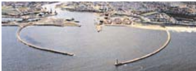
Entrance to the River Wear (Sunderland)
