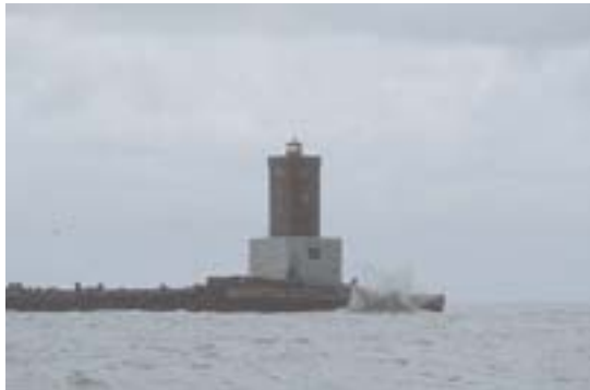
Minsener Oog Disused Light Tower (Buhne A)
