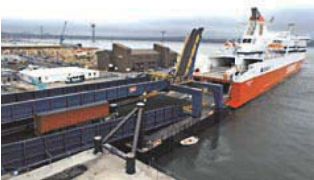
Rosyth Ferry Terminal
