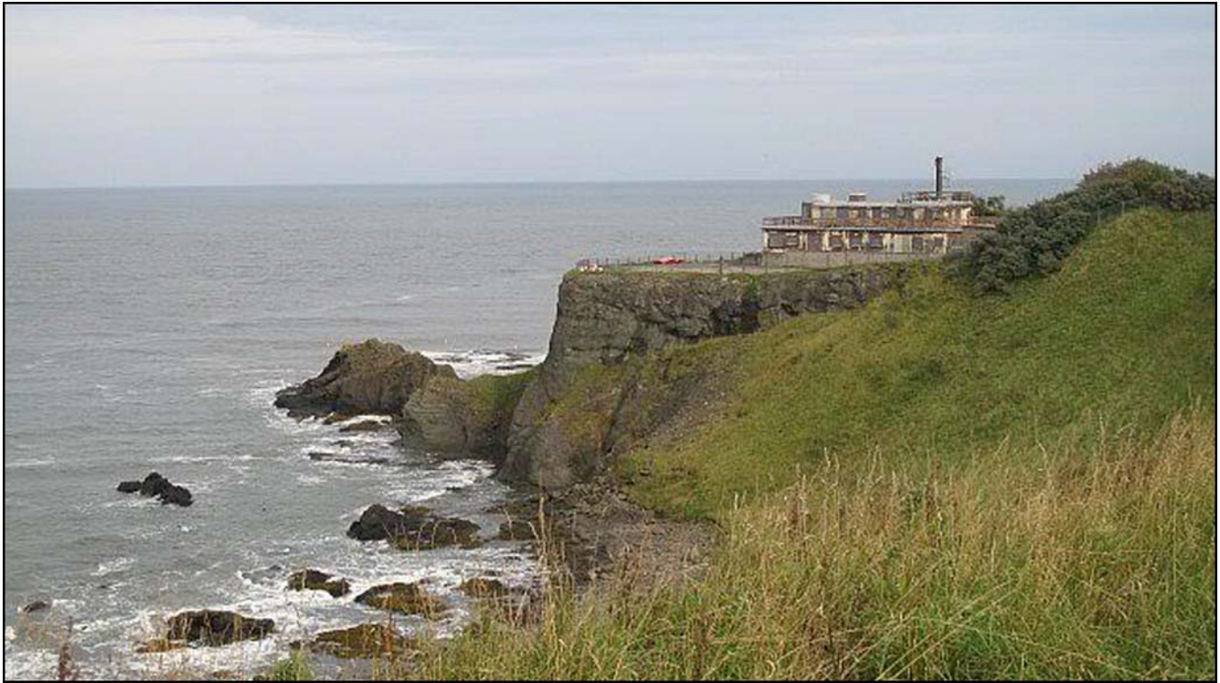
Ginhead stack and buildings
