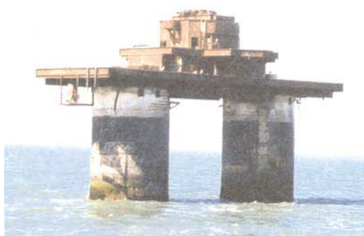
Knock John Tower
