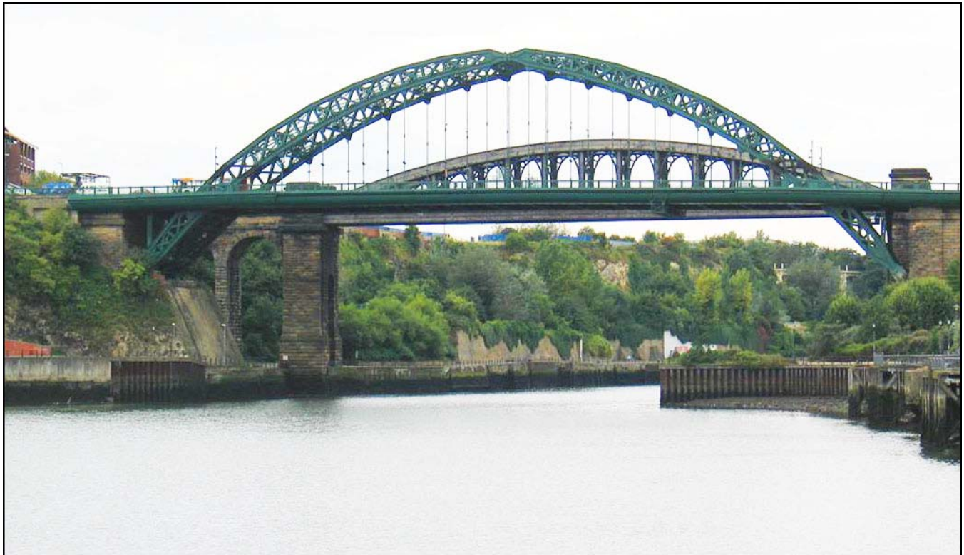
Sunderland Railway Bridge
