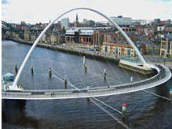
Gateshead Millennium Bridge (closed)
