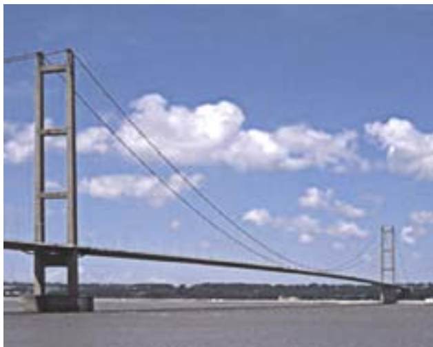
The Humber Bridge
