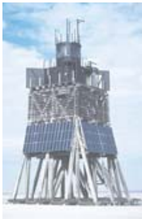
Suderoogsand Light (Refuge Beacon)
