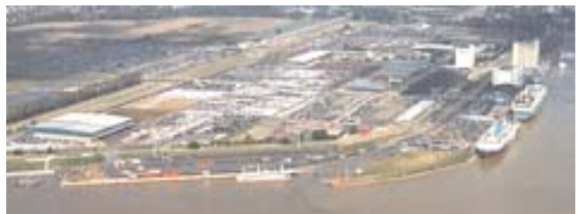
Emden Ro-Ro Terminal
