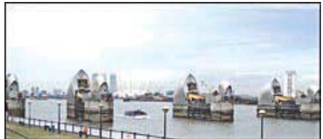
Thames Tidal Barrier
