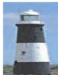
Spurn Head Lighthouse (disused)
