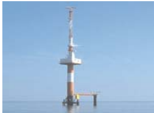
Hooksielplate Radar Tower
