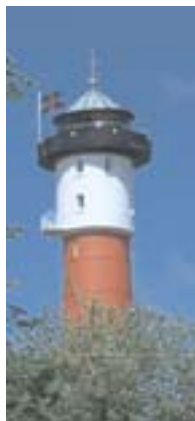
Wangerooge Disused Light Tower
