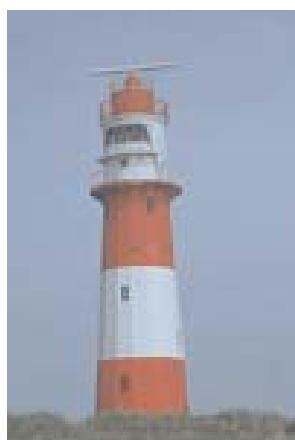
Borkum Little Disused Light Tower
