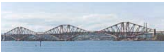
The Forth Bridges from NE
