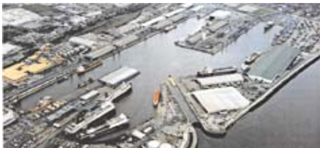
Hull—King George Dock and Queen Elizabeth Dock
