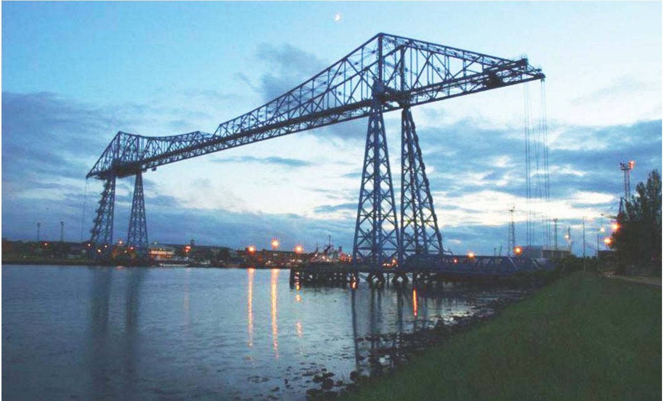
Tees Transporter Bridge
