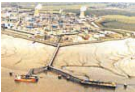
Salt End Oil Terminal
