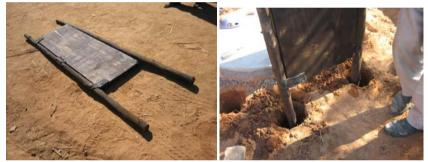
Fitting a car rubber hinge to one of the treated gum poles. The final pole and door unit ready to mount in front of the slab. The two holes drilled for the two main "king posts" are drilled in front of the slab. The door should be about 65cm in front of the squat hole and door posts 50cm apart.
