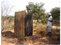
A series of hardwood or treated poles has been placed around the slab in holes drilled by an earth auger. Three wires have been tightly wrapped around the holes for attachment of the cleaned grass. The grass is attached to the poles as bundles. A disc of strong concrete can be made to fit over the ventilation pipe hole before a pipe is fitted. A vent pipe can be fitted later
