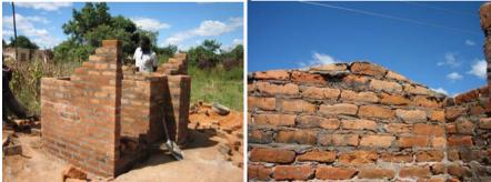
The walls are built up. The end walls and mid wall which will support the roof are built up so the roof will slope outwards.
