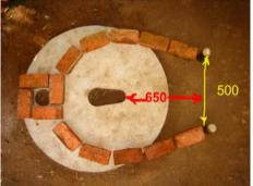
The distances between poles (500mm) and between the door and the squat hole (650mm)
