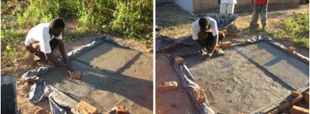
A sheet of plastic is best laid on the ground to cover the soil within the brick mould. The cement will loose less moisture when laid over plastic and will develop more strength. The mix of cement is laid in sections. The mix of cement is 4 parts river sand to 1 part PC15 cement. To make the roof 3 mixes of 12li cement and 48li river sand (4:1) were used.
