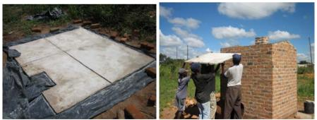
The four panels are allowed to cure for at least 7 days being kept wet at all times. Each panel is carefully lifted from the plastic sheet and placed on the superstructure in the appropriate place, embedded in cement mortar.
