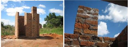
The vent pipe is raised 6 courses above the wall level. Later it is fitted with a corrosion resistant fly screen.
