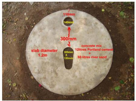
Details of concrete slab for uBVIP
