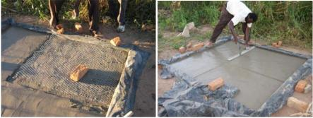
Each section is covered with a layer of cement about 20mm thick and the wire is laid over this to cover the section. The wire is then covered with another layer of cement. Later on the concrete will be cut with a trowel when still soft. The sections of wire in the concrete must be separated clearly so the trowel cuts through concrete only. The concrete is then covered for the night. It is watered the following morning and kept wet and covered for a week before moving on to the structure.
