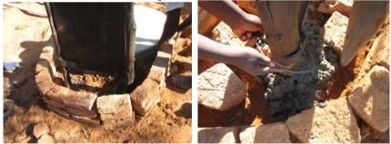
A mould made of bricks is built up around the two main poles. This is filled with a mix of broken bricks, stones and concrete to anchor the posts. Each post is surrounded by a ring of steel wire.
