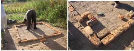
An area of ground is levelled and a mould made with bricks to suit the size of the roof required. In this case the total area was 2m X 1.8m.The chicken is laid within the mould and cut up into four pieces (900mm x 870mm (2 pieces) and 900mm x 1130mm (2 pieces). The exact measurements should be taken from the structure, which varies slightly in each case. A recess was made in one of the four panels for the vent pipe.
