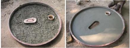
Making the concrete slab for the uBVIP. Half the concrete mix is added first. Then the wire reinforcing is added. Then the remainder of the concrete is added and smoothed down flat.
