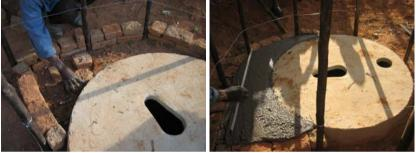
Poles are placed around the slab in a spiral shape. Cement left over from the pit lining is used to make a cement floor in front of the slab. This cement can be extended into the entrance of the toilet
