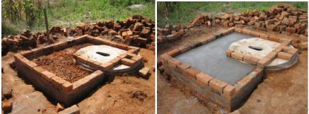
The brick walls are laid on the foundation so the outer dimensions of the brick walls are close to 1.45m X 1.85m. The walls are built up to slab level. The toilet floor area is then backfilled with brick rubble to lower slab level. This is then filled with a concrete mix (10 litres cement + 50 litres river sand).
