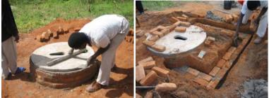
The slab is made level on the elevated brickwork above ground level and the weak cement mortar smoothed down around the slab so the slab and brick lining are airtight. The slab and pit must have an airtight fit of the vent pipe is to work properly. A trench is cut down in the soil around the toilet. The brick foundation for the walls will be laid in this following the dimensions below,
