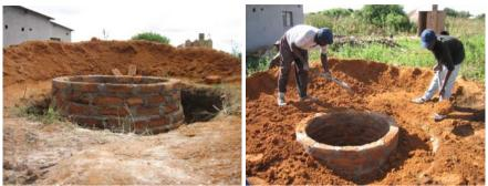
The pit lining extends about 20cm above ground level. The annular space between the dug pit and the pit lining being filled in.
