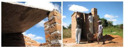
Each panel is supported by the dividing wall in the centre of the structure as shown
