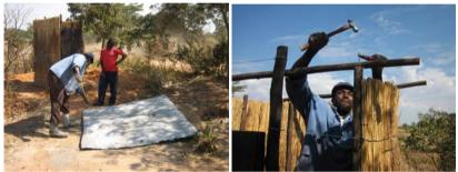
The roof is prepared for attachment to the grass and pole structure. Extra poles are added to the upright poles for attachment to the roof.
