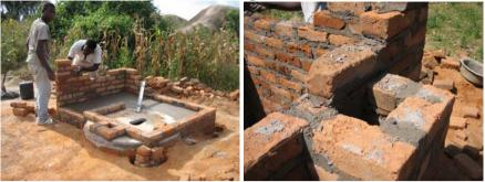
Walls and vent come up together. The walls are built up to 1.8m in height and the pipe to about 2.4m, The internal surfaces of the brickwork inside the pipe must be kept smooth.
