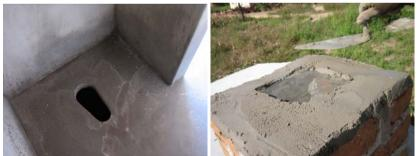
All the internal surfaces of the Blair VIP are plastered. The floor is also dished to allow drainage of water into the brick lined pit. A fly screen made of aluminium is then embedded in cement mortar to the top of the vent pipe
