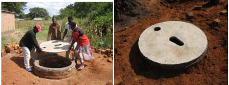
Weak mortar is laid around the rim of the pit lining. The slab is then mounted. The orientation of the slab depends on the type of structure to be built. In this case a square spiral structure will be built, so the pipe hole will be on the same side as the toilet structure opening.
