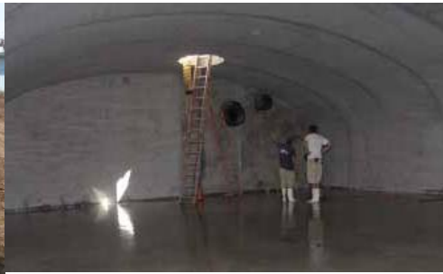
Photo 5: Inside view of an empty low flow-diversion chamber (Pirazzi)
