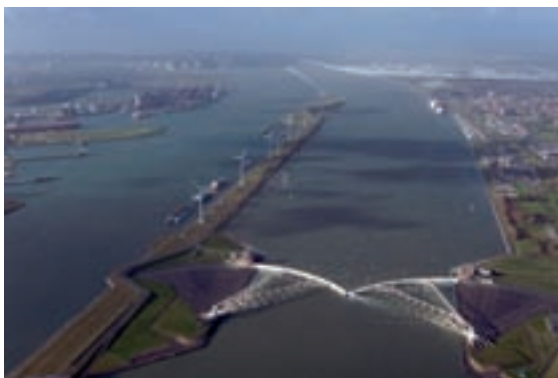
Figure 95. The Maeslantkering is a storm surge barrier in the Netherlands, which automatically closes when needed for protection. It is part of the Delta Works and it is one of largest moving structures on Earth. (©AeroLinphoto, the Netherlands)
