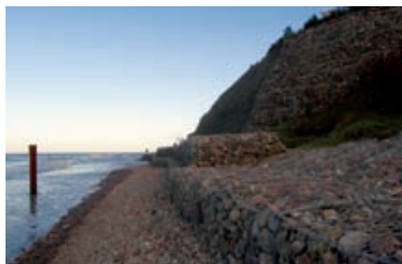
Figure 7. Protection of cliffs against erosion by geotextile and gabion structures in Gdansk, Poland. (©Simon Claus for the EU FP7 Project THESEUS)
