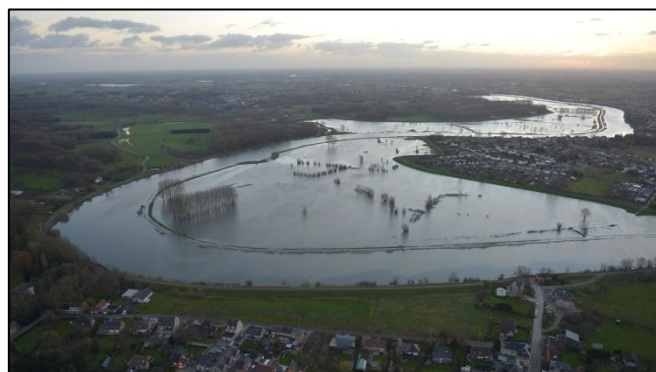
Figure 4. FCA/CRT 'Bergenmeersen' filled during storm surge of 6 th of December 2013.
