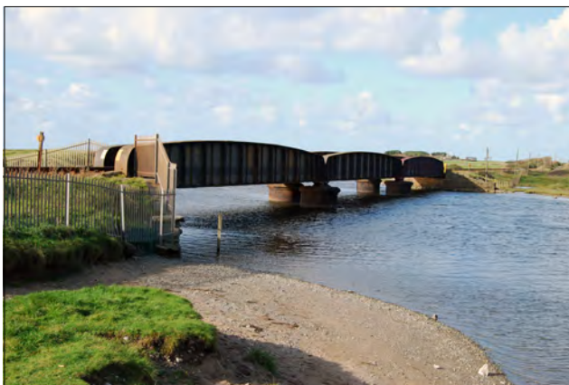
Railway bridge built in 1911 across the Dysynni.
