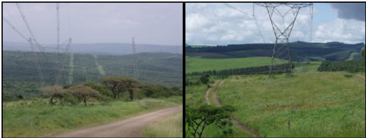
Figure 8-2: View of existing power lines in the study area.
