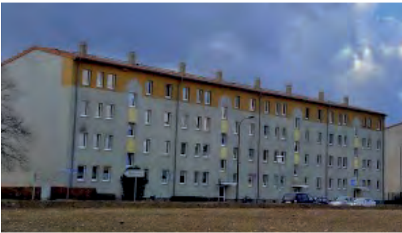
Zeilenbau in Gransee 5
