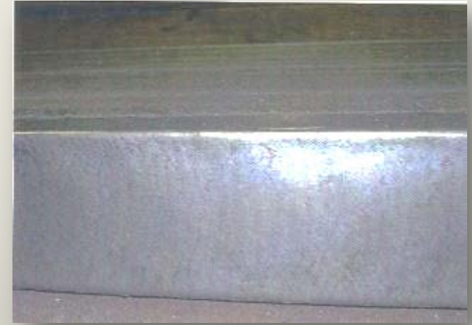
Typical slab surface and edge scarfed by Evertz – MFA-HB 009h
