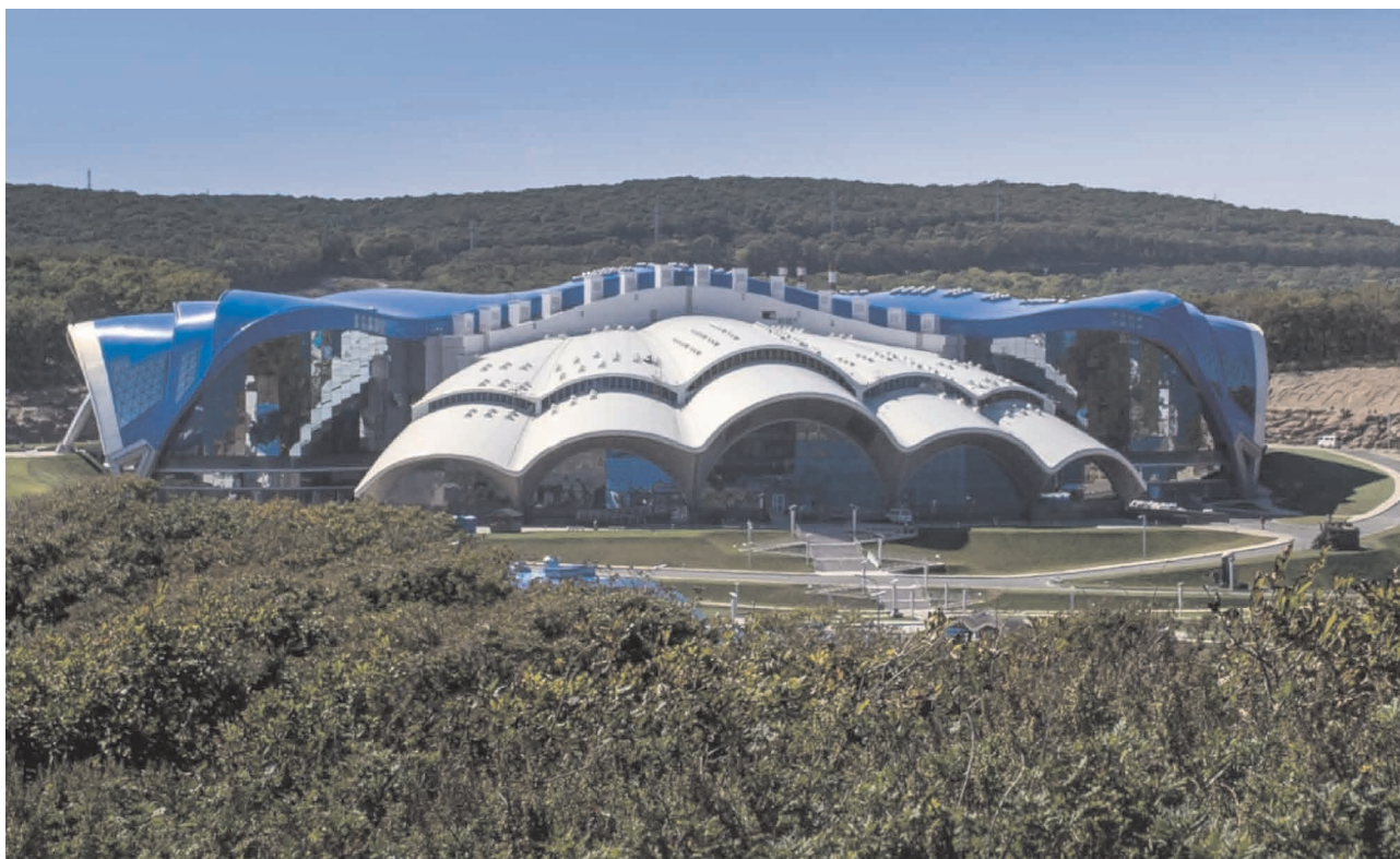
Fig. 1. Main building of the Primorsky Aquarium FEB RAS.
