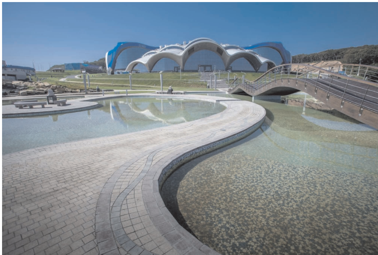
Fig. 2. The promenade area side view of the Primorsky Aquarium FEB RAS main building.
