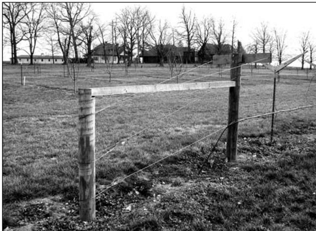
Fig. 6-5. Single span brace assembly
