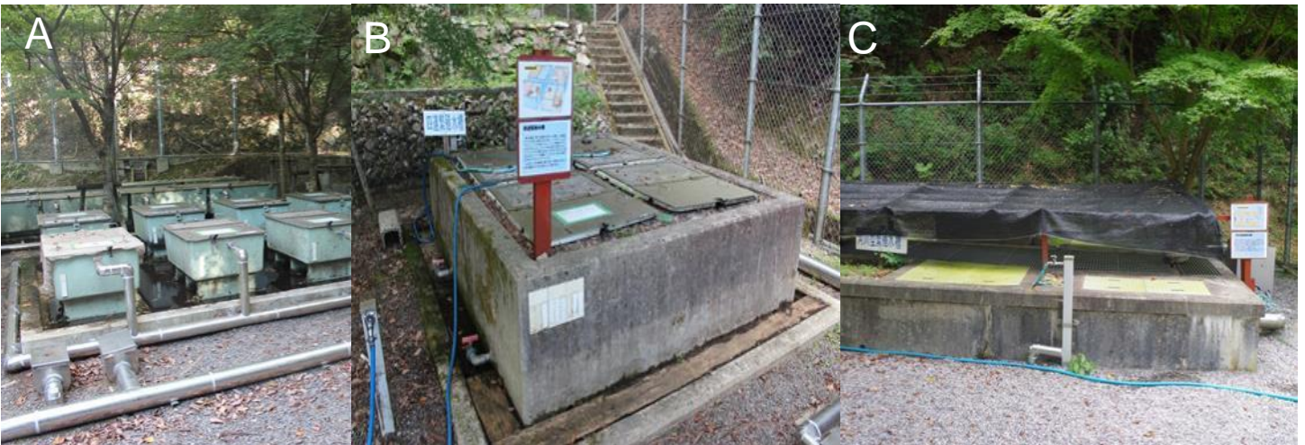
Figure 37. A. Water supply goes into each tank individually. B. Four connective breeding tanks. C. Stream type breeding tank. Image: Yuki Taguchi.
