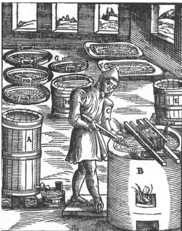
Pans and tubs for crystallisation – from Ercker.
