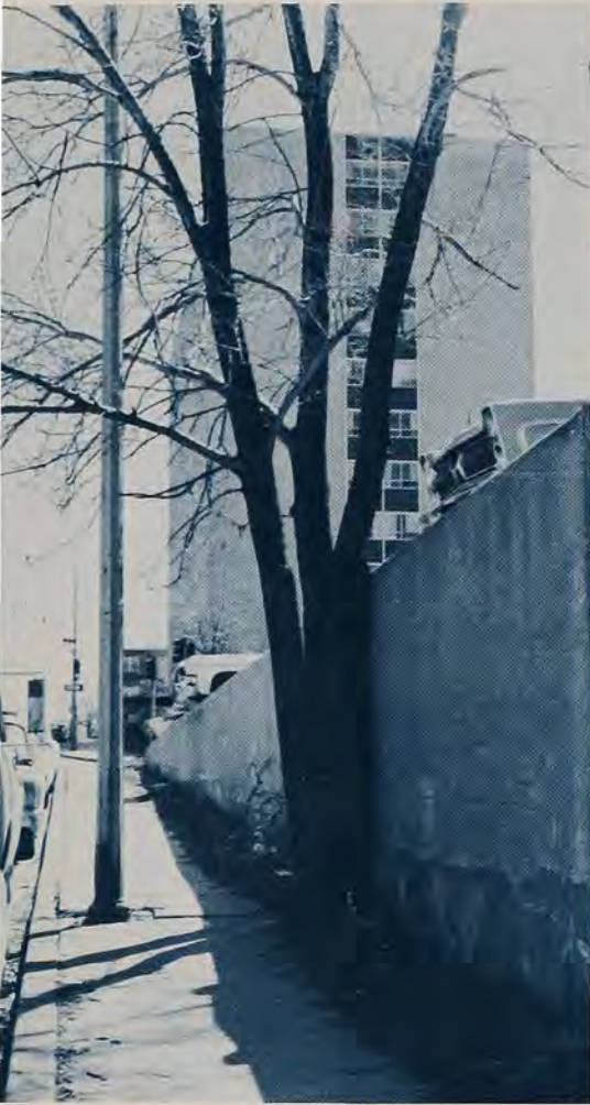
Something will have to give; the sidewalk, the retaining wall, or, less likely, the volunteer elm. Cut back once, as indicated by multiple trunks, it apparently is there to stay.
