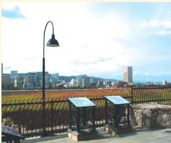
The Multnomah County Green Roof public plaza in Portland.
