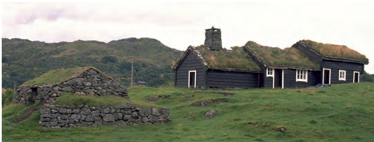
Photo 10.8. Bogatunet, Radøy. A long house divided into four rooms with different functions: a workshop with a loft, a room with open fire, a room for smoking fish and meat and a living room, as was typical of many 18th and 19th century farms. Photo: Helge Sunde.
