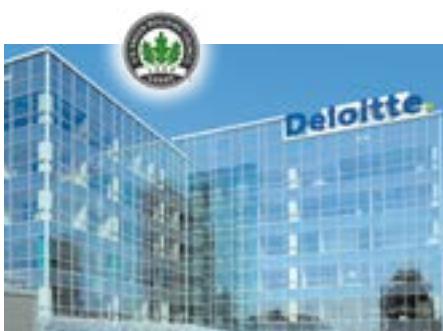
Acrum City, Varšava – LEED PLATINUM
