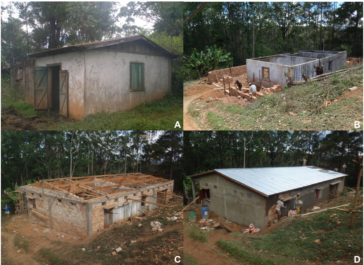
Figure 1. The facility was constructed between November 2010 and March 2011 from the foundations of an old abandoned forest station. A) Original abandoned building in January 2009. B) Facility construction November 2010. C) Facility construction December 2010. D) Facility construction January 2011.
