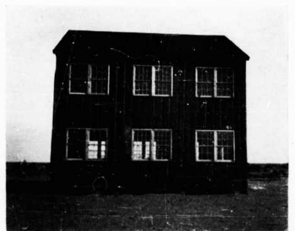
FIGURE 162. West elevation of Barracks 3 after Test 3
