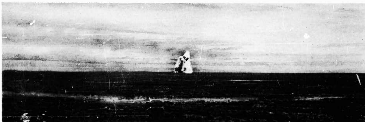
FIGURE 197. Explosion of Revetment 2, 1st stage
