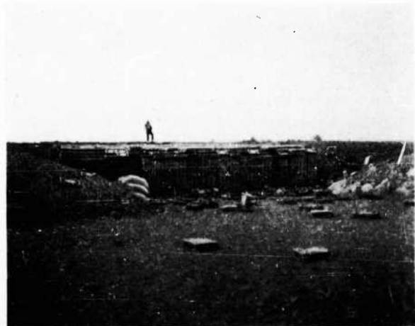
FIGURE 53. Front of Revetment 2 after Test 1
