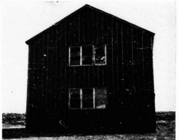
FIGURE 114. North elevation of Barracks 3 after Test 2
