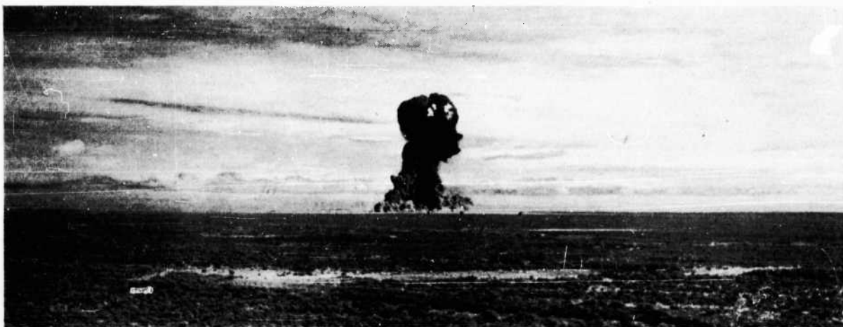
FIGURE 198. Explosion of Revetment 2, 2nd stage
