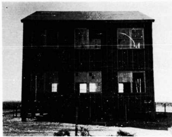
FIGURE 59. East elevation of Barracks 2 after Test 1
