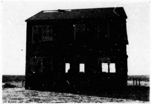
FIGURE 108. East elevation of Barracks 1 after Test 2
