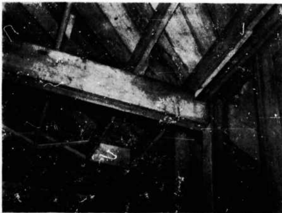
FIGURE 120. Displacement of south wall and column supporting 2nd floor, ground floor, Barracks 1 after Test 2
