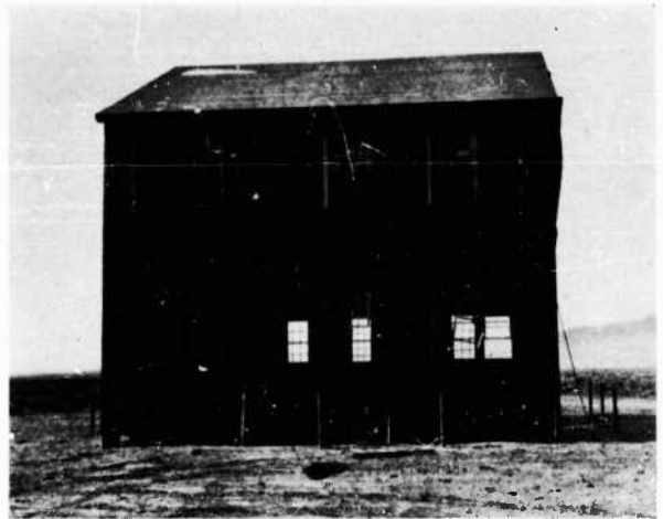
FIGURE 55. East elevation of Barracks 1 after Test 1
