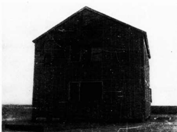
FIGURE 187. Barracks 2 after Test 4; north elevation
