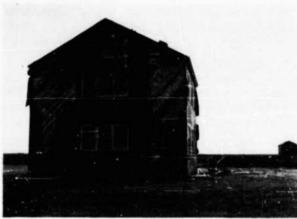
FIGURE 151. North elevation of Barracks 1 after Test 3
