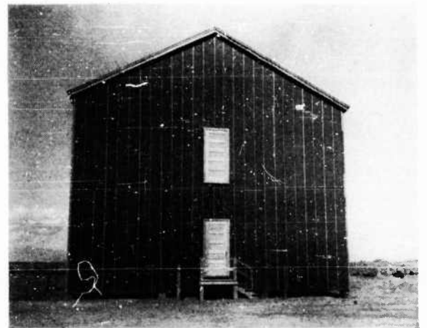
FIGURE 57. South elevation of Barracks 1 after Test 1
