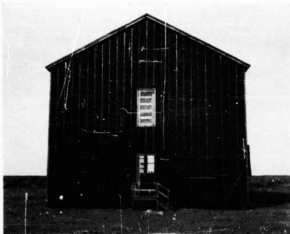
FIGURE 161. South elevation of Barracks 3 after Test 3
