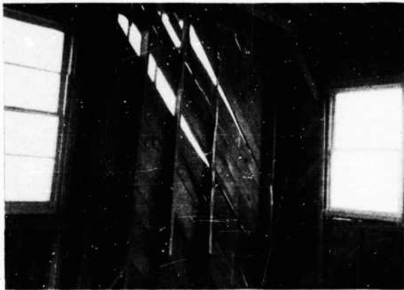
FIGURE 165. Interior, Barracks 1 after Test 3, showing condition of northeast corner, 2nd story
