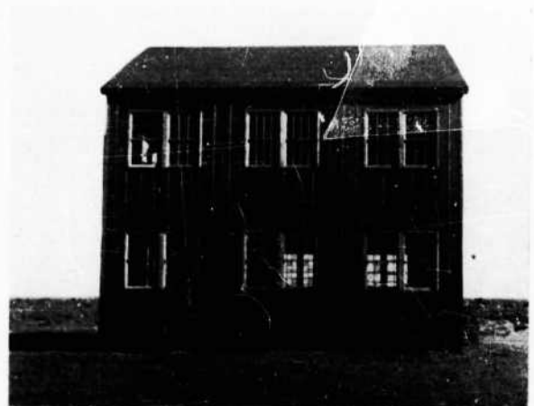
FIGURE 215. West elevation of Barracks 3 after Test 5
