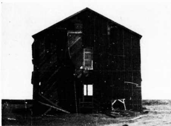
FIGURE 185. Barracks 1 after Test 4; south elevation
