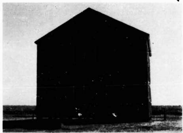
FIGURE 110. North elevation of Barracks 2 after Test 2
