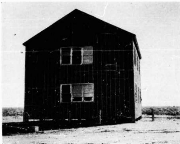
FIGURE 58. North elevation of Barracks 2 after Test 1
