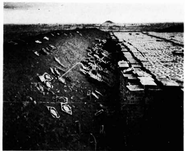
FIGURE 51. Revetment 1 after Test 1. Looking north along edge of mine stack from southwest corner
