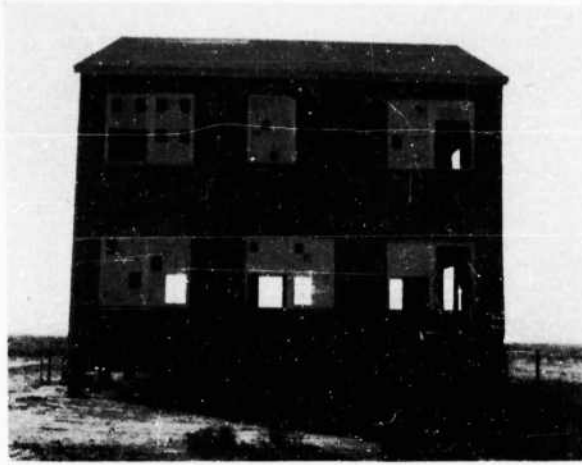
FIGURE 111. East elevation of Barracks 2 after Test 2
