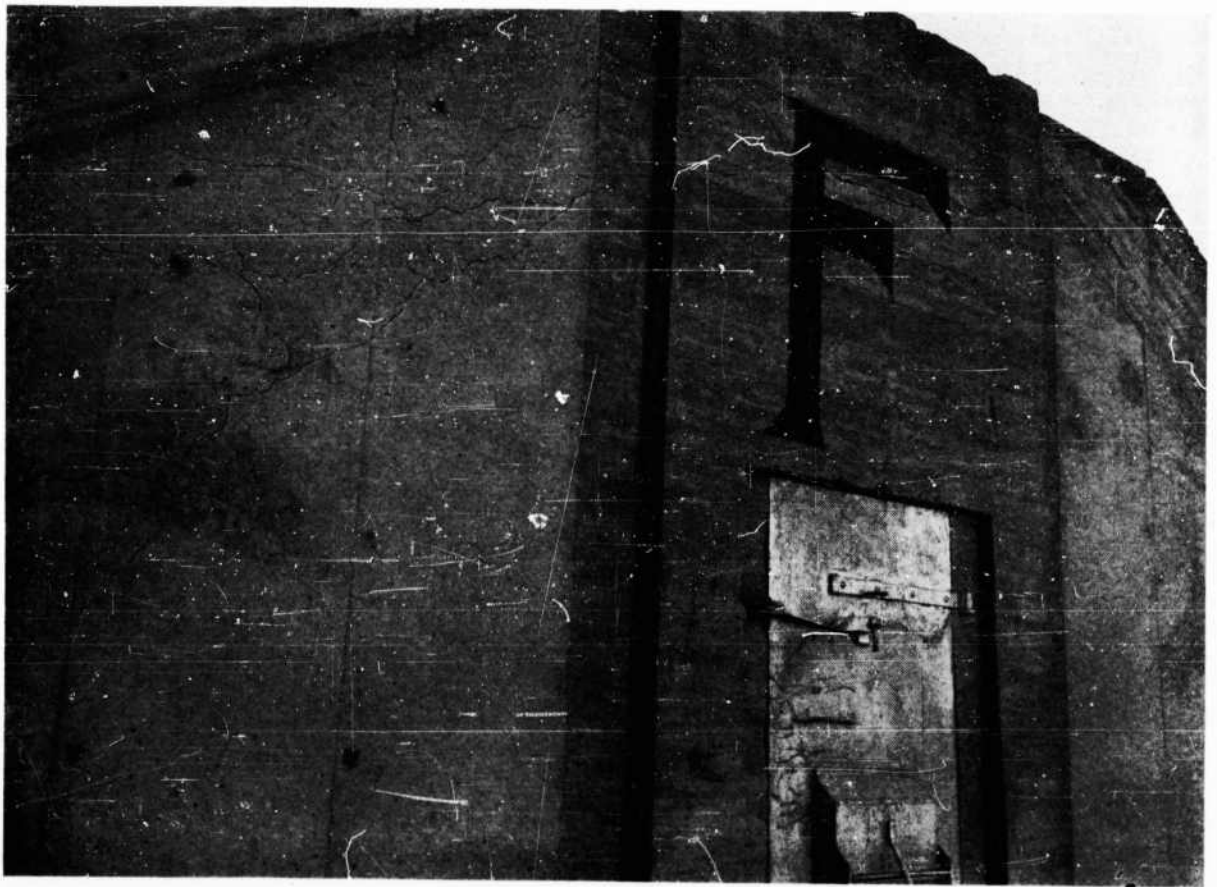
FIGURE 48. Close-up of front of Igloo F after Test 1
