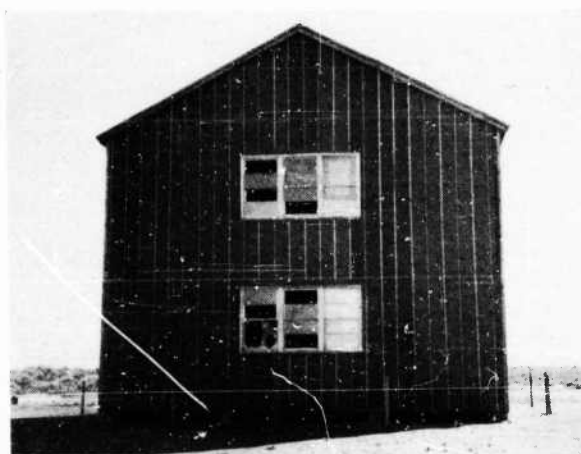
FIGURE 60. North elevation of Barracks 3 after Test 1
