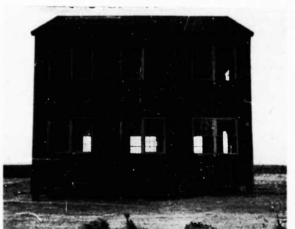
FIGURE 156. East elevation of Barracks 2 after Test 3
