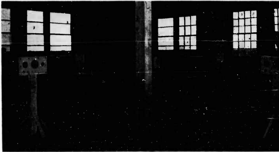
FIGURE 129. Interior of lower story, looking northeast, Barracks 3 after Test 2
