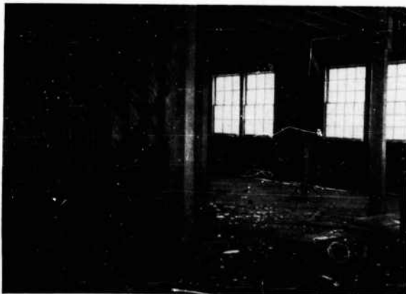
FIGURE 66. Interior of Barracks 1 after Test 1. Second floor, looking southwest
