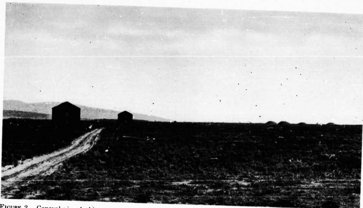
FIGURE 2. General view looking north toward explosion area, showing Barracks 1 and 2 to left and igloos on right.
