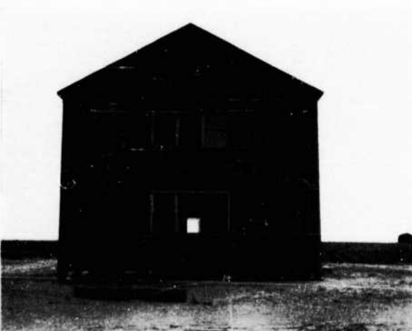
FIGURE 155. North elevation of Barracks 2 after Test 3
