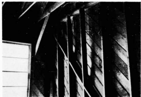
FIGURE 73. Interior, Barracks 2 after Test 1. Second story, northwest corner, showing displaced and fractured studding
