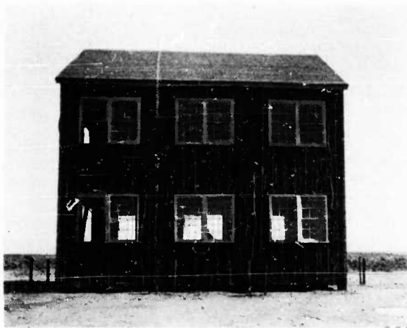
FIGURE 56. West elevation of Barracks 1 after Test 1
