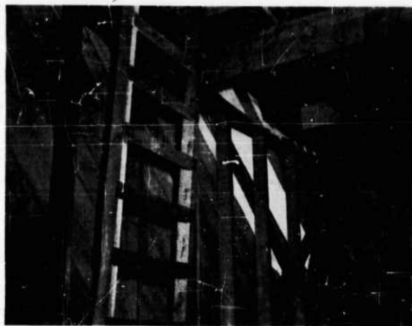
FIGURE 196. Interior of Barracks 1 after Test 4, showing separation of south wall from second floor, and missing sheathing
