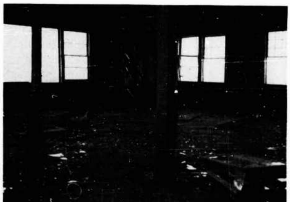
FIGURE 67. Interior of Barracks 1 after Test 1. Second floor, looking northeast
