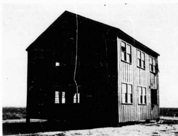
FIGURE 208. North elevation of Barracks 2 after Test 5
