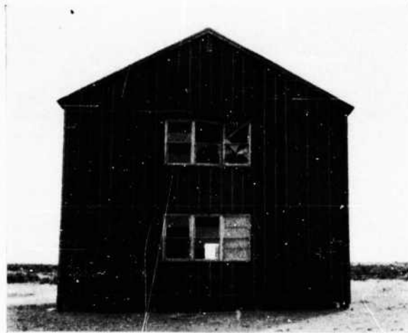
FIGURE 159. North elevation of Barracks 3 after Test 3
