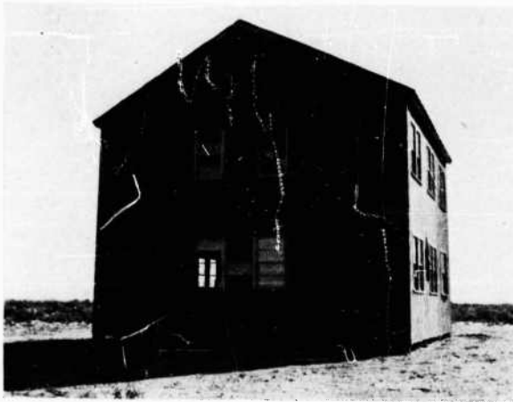
FIGURE 212. North elevation of Barracks 3 after Test 5
