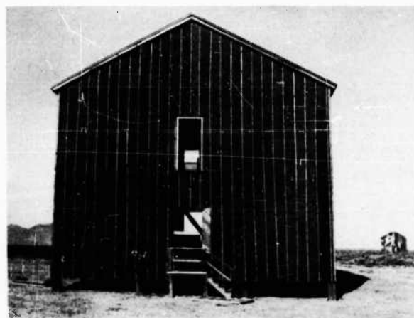
FIGURE 210. South elevation of Barracks 2 after Test 5
