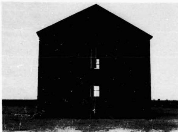
FIGURE 157. South elevation of Barracks 2 after Test 3
