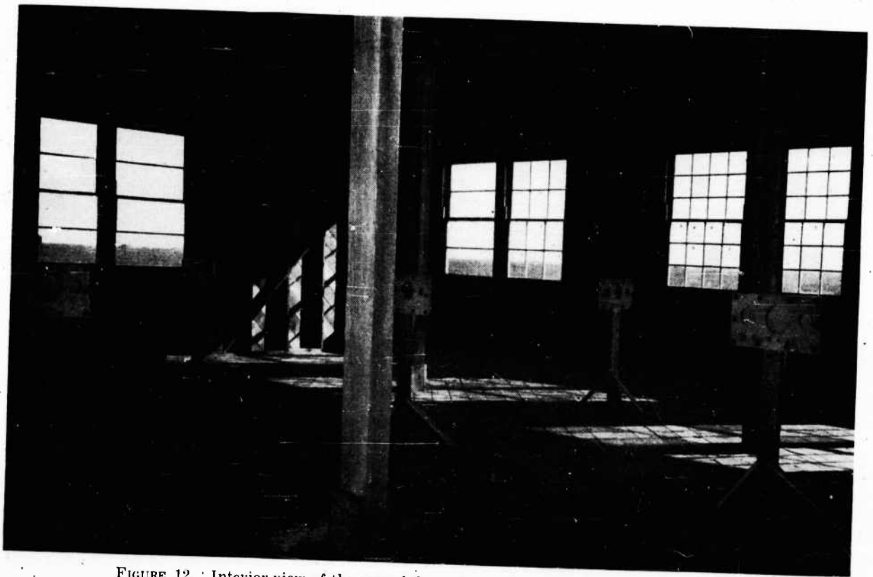
FIGURE 12. Interior view of the second floor of one of the barracks, looking northeast
