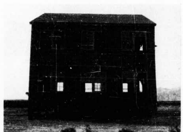
FIGURE 188. Barracks 2 after Test 4; east elevation
