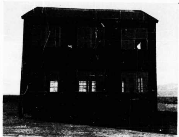
FIGURE 192. Barracks 3 after Test 4; east elevation
