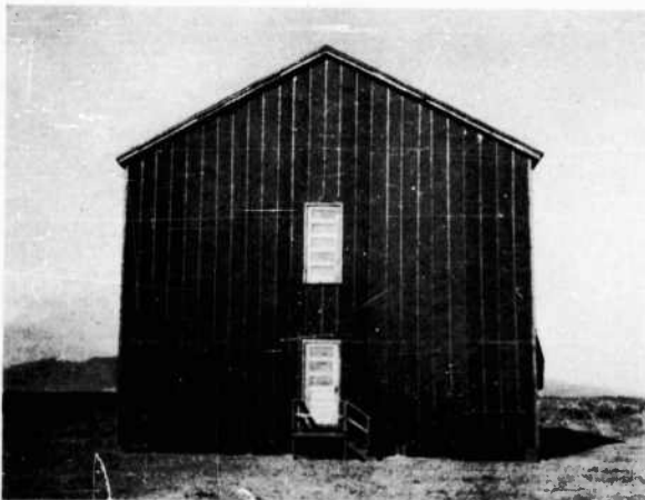
FIGURE 214. South elevation of Barracks 3 after Test 5
