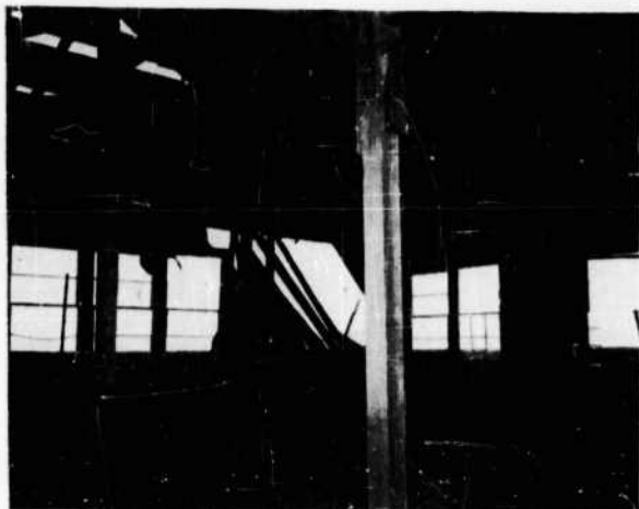
FIGURE 195. Interior of Barracks 1 after Test 4, looking toward northeast corner on second floor
