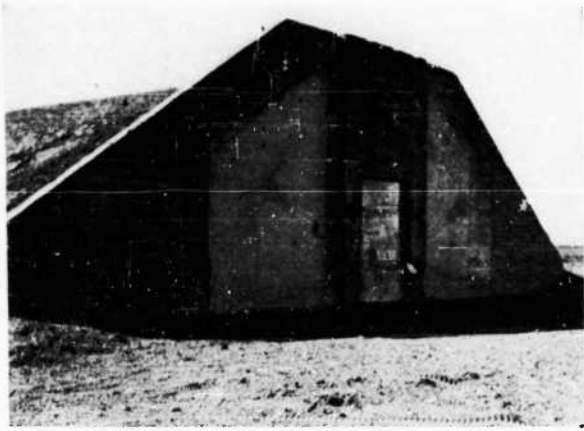
FIGURE 97. Front of Igloo F after Test 2
