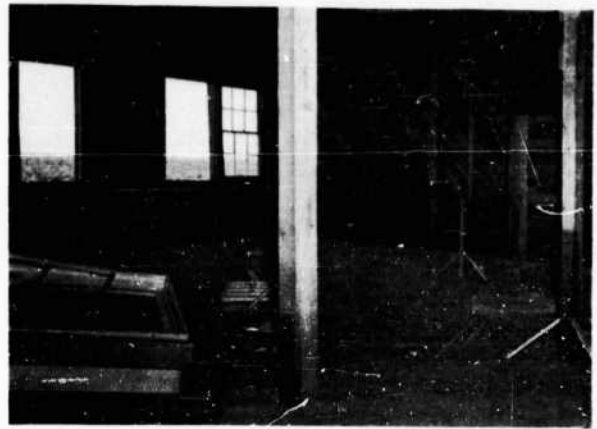
FIGURE 63. Interior of Barracks 1 after Test 1. Ground floor, looking southeast
