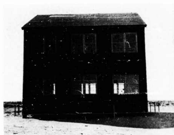
FIGURE 61. East elevation of Barracks 3 after Test 1
