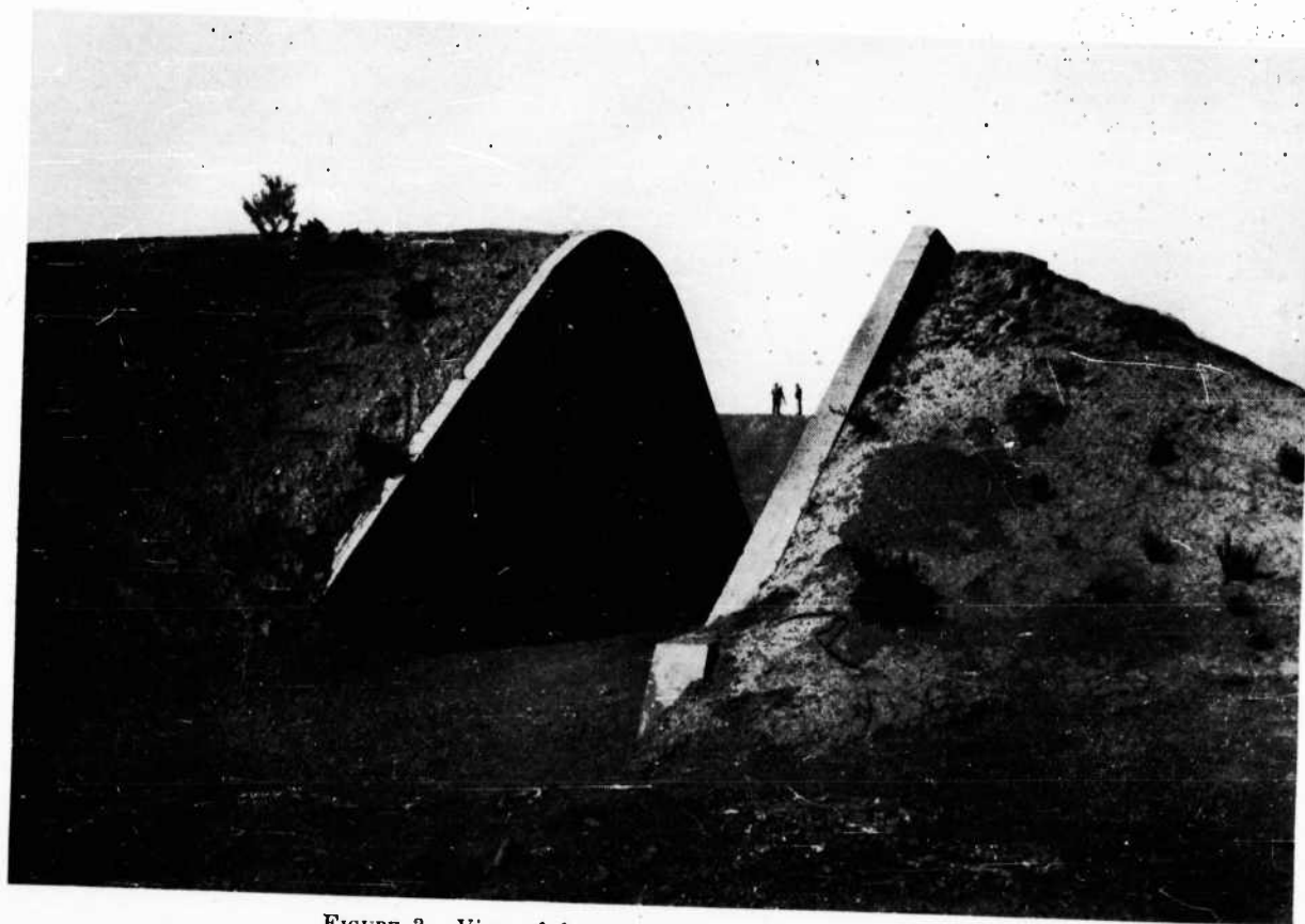
FIGURE 3. View of front end and door barricade, Igloo D
