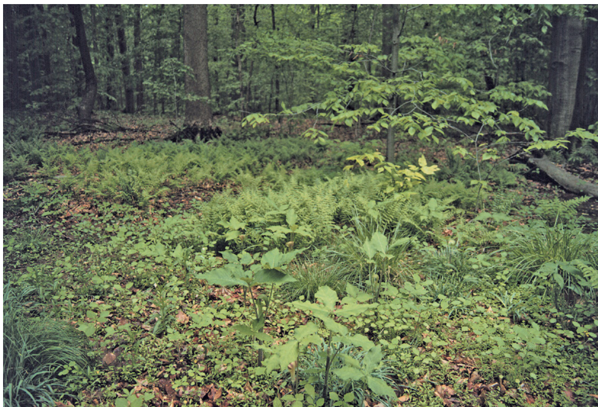
In one of the project's woodland construction zones native plants including wildflowers, ferns, and sedges can be seen one year after pipeline installation.
