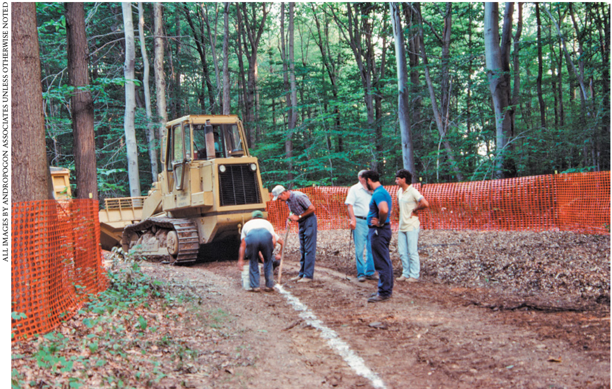
Loantaka Brook Reservation, Morristown, New Jersey, contains diverse plant communities including several forest and meadow types. To limit ecological disruption, a natural gas pipeline installed through the reservation in 1986 was carefully routed and constructed. Here, the pipeline alignment is being marked.
