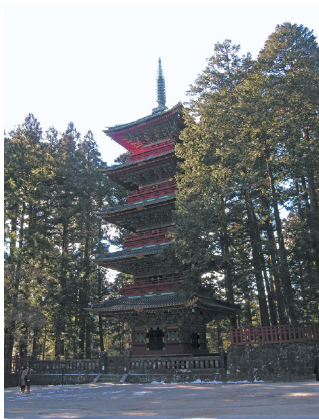
Photograph from the same position as that of the left photograph on January 13, 2007.
