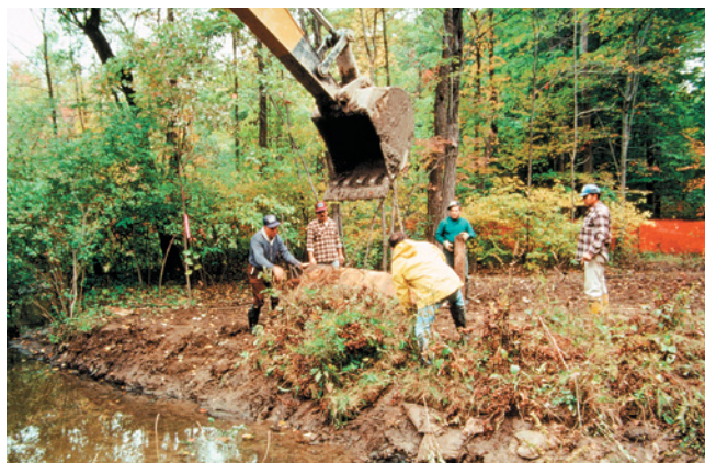
To preserve existing native plants and seedbanks, soil blocks were carefully lifted in advance of the construction trench, then relaid at the back of the line where the trench had been refilled. Seen here, soil blocks from the wet meadow are moved and temporarily stored (left), and later transplanted (right).
