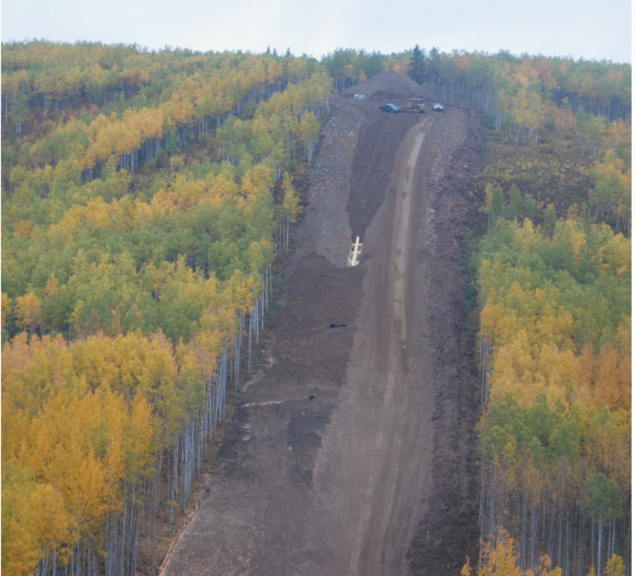
Typical pipeline construction involves clearcutting and environmental disruption of wide swaths of land. This photograph shows installation of a natural gas pipeline in northeastern British Columbia.
