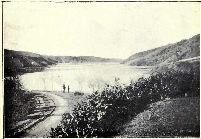
RATHMINES WATERWORKS—THE LOWER RESERVOIR.
