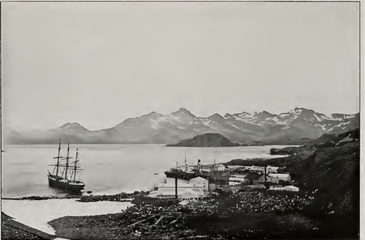
FIG. 2.—Whale Factory, Leith Harbour, South Georgia.
