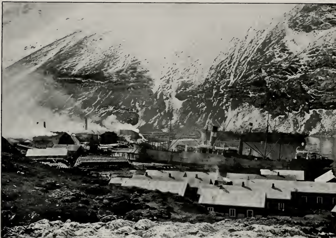
FIG. 1.—Whale Factory, Leith Harbour, South Georgia.
