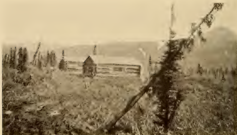
FIG. 64.—Contractors' cabins on the line of the government railroad near Broad Pass, Alaska.
