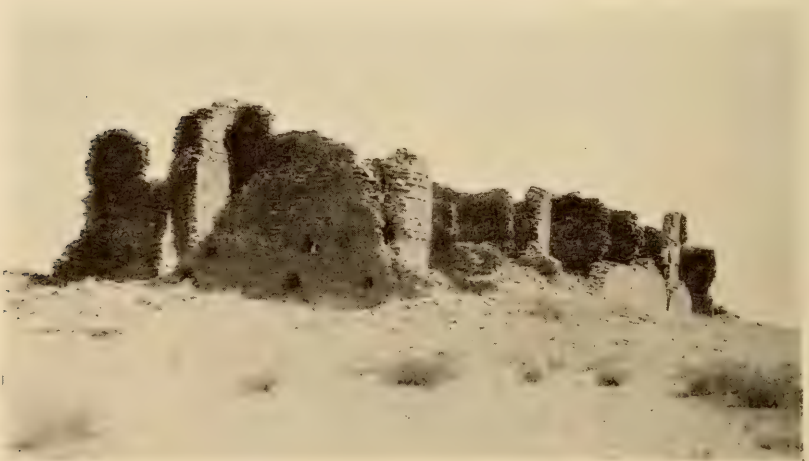
FIG. 119.—Part of Pueblo Pintado, as seen from the northwest. This ruin was visited by Lt. J. H. Simpson, August 26, 1849, on his memorable advance into the Navaho country; the large timbers noted by Simpson and other early explorers have since been torn from the walls, causing obvious destruction to the latter.
