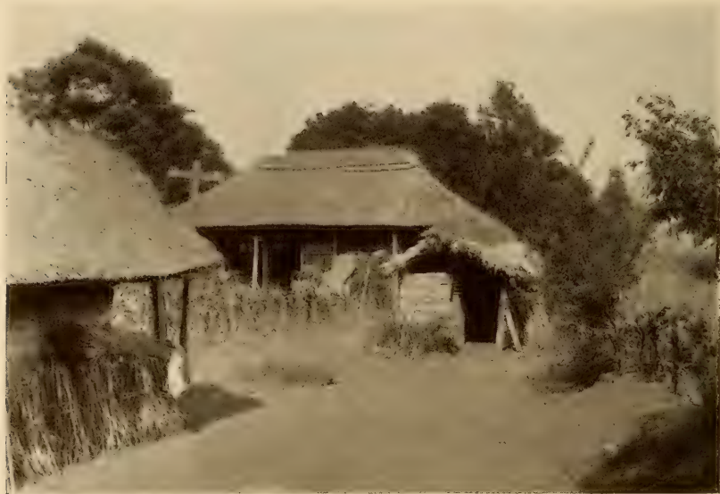
FIG. 34.—A peasant's hut near Gotemba, Japan. The roofs of the building are thatched with coarse grass. The bundles are for firewood.
