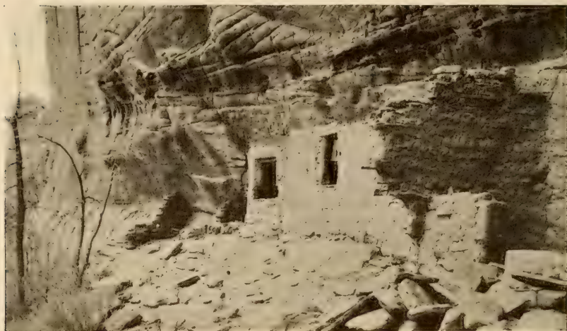
FIG. 113.—Part of a cliff village in a cave on the east side of Cottonwood Canyon, near Kanab, Utah. The village includes nineteen rooms and a nearby spring furnished excellent water for the ancient inhabitants.
