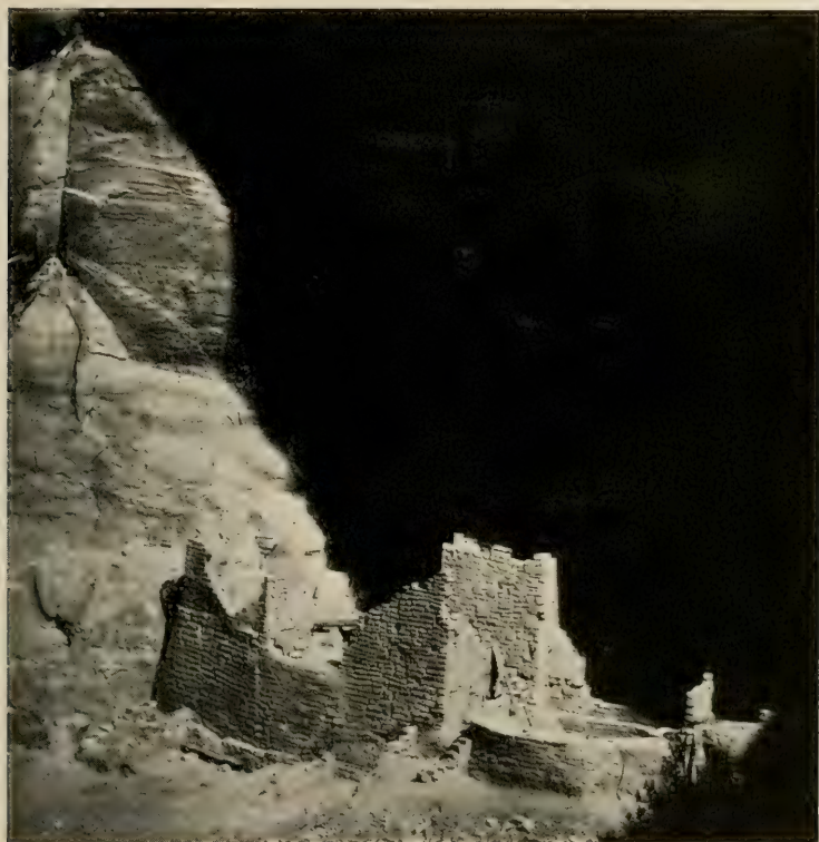
FIG. 57.—Western end of Square Tower House, excavated and repaired. Photograph by Fewkes.
