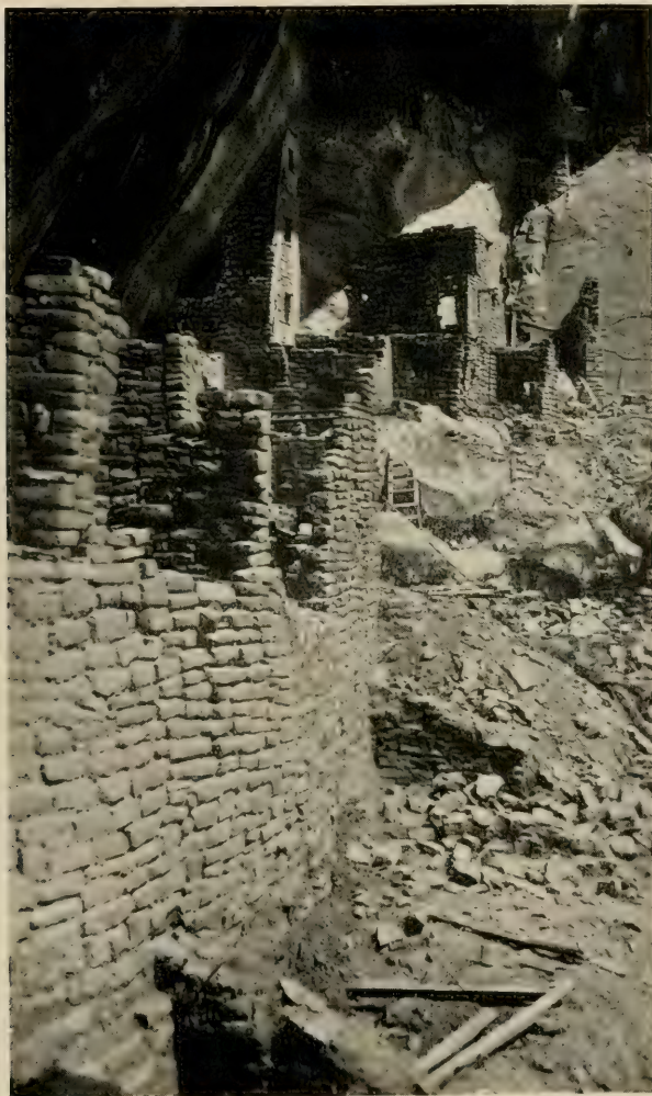
FIG. 50.—View of Square Tower House from the west, before excavation and repair. Photograph by Fred Jeep.
