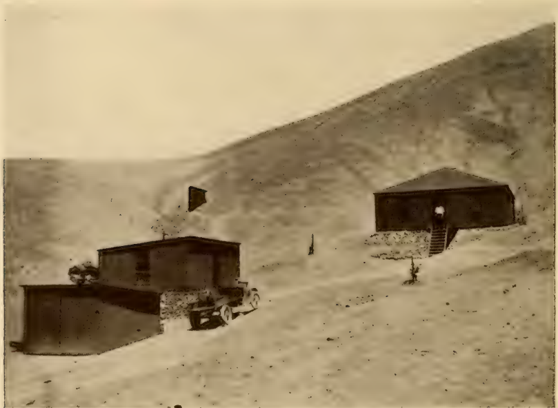
FIG. 32.—Garage, Shop and Dwelling, Mount Montezuma.
