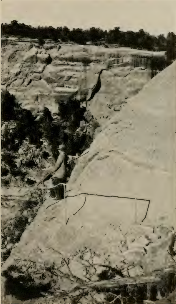
FIG. 48.—The footpath blasted in the cliff at the most difficult part of the ancient trail where the tourists are represented in figure 47. Photograph by Fred Jeep.
