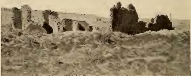
FIG. 115.—The north wall of Pueblo Bonito, viewed from the northeast. This is the largest and justly the most famous of all the Chaco Canyon ruins; it covers nearly three acres of ground and some of its walls still stand to a height of forty feet. When occupied Pueblo Bonito probably contained as many as 800 rooms, sheltering over 1200 individuals.
