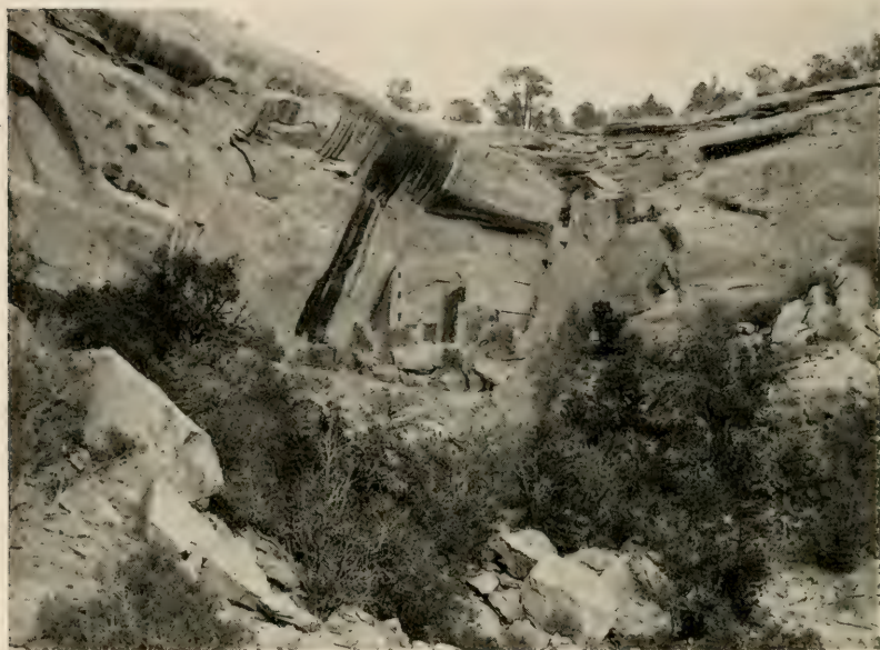
FIG. 65.—Square Tower House repaired, as seen from the west. Photograph by T. G. Lemmon.
