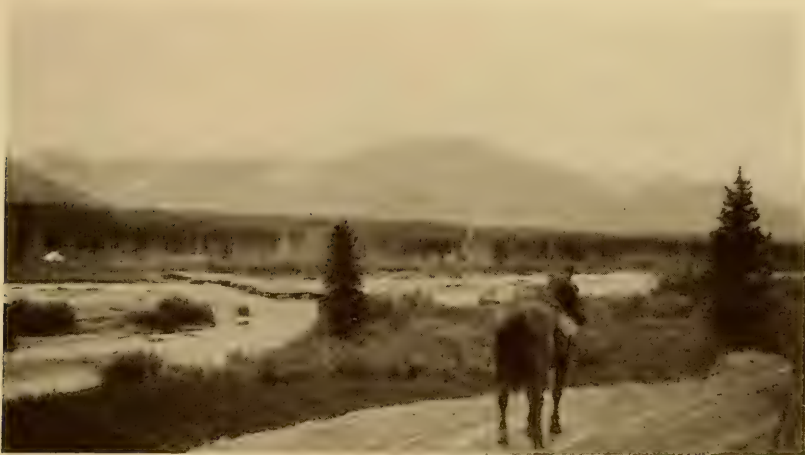
FIG. 63.—Middle fork of Chulitna, a little south of Broad Pass. Corduroy bridge of the Alaskan Engineering Commission.
