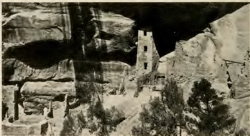
FIG. 52.—View of the Tower completely repaired. Photograph by Fred Jeep.
