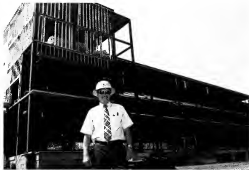
Tony Carter '61 is overseeing the construction of the Center for Marine Science Research at Myrtle Grove, which is scheduled for completion in summer 1999. Ground was broken for the student recreation center in May, and construction is now underway. That 64,000-square-foot building near Wagoner Hall should be complete in time for the start of classes in fall 1999. An $8.4 million classroom building, to be located near Morton Hall, is in the design stage and should be built by April 2000.
