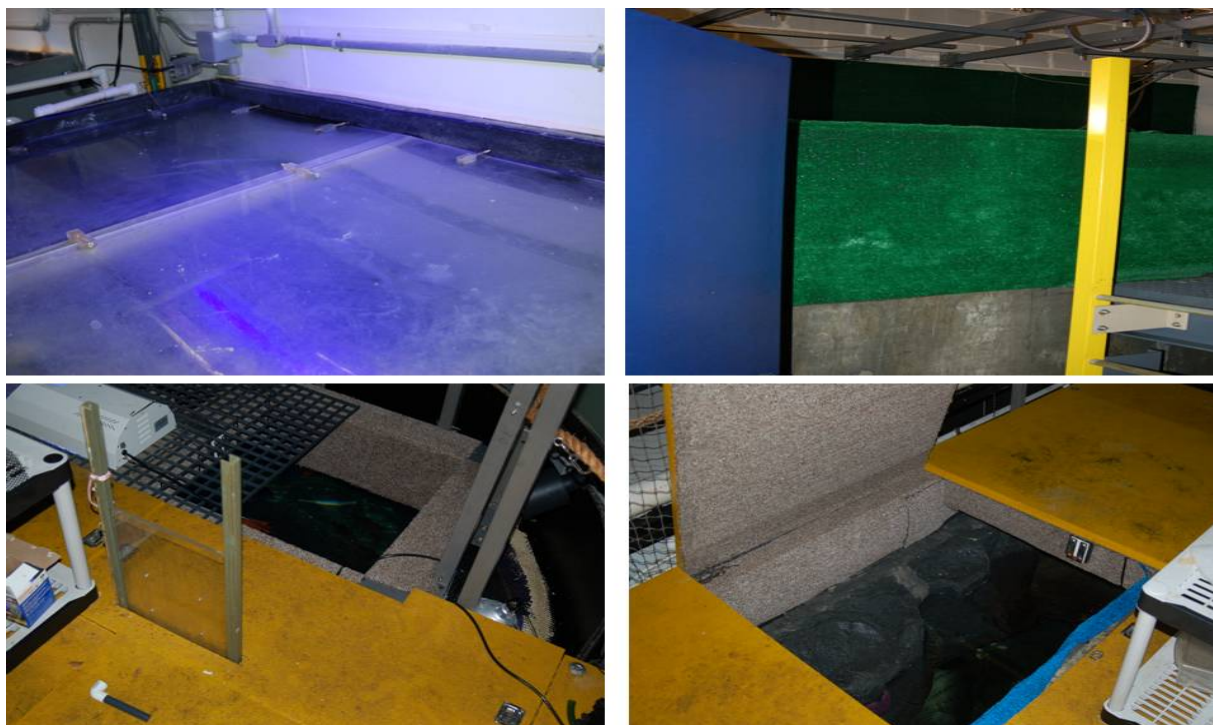
Figure 10. Containment strategies for octopus exhibits. Top left: A 2-piece acrylic lid with stainless steel latches. Top right: A tank with extensive AstroTurf on the lip and down the sides to prevent octopods from being able to grip the surfaces. Bottom: A GPO tank. Note structural beams and tank struts covered with AstroTurf, and acrylic shift doors (left). At right, note the fiberglass lid with all internal surfaces coated in AstroTurf. Photos courtesy of B. Christie
