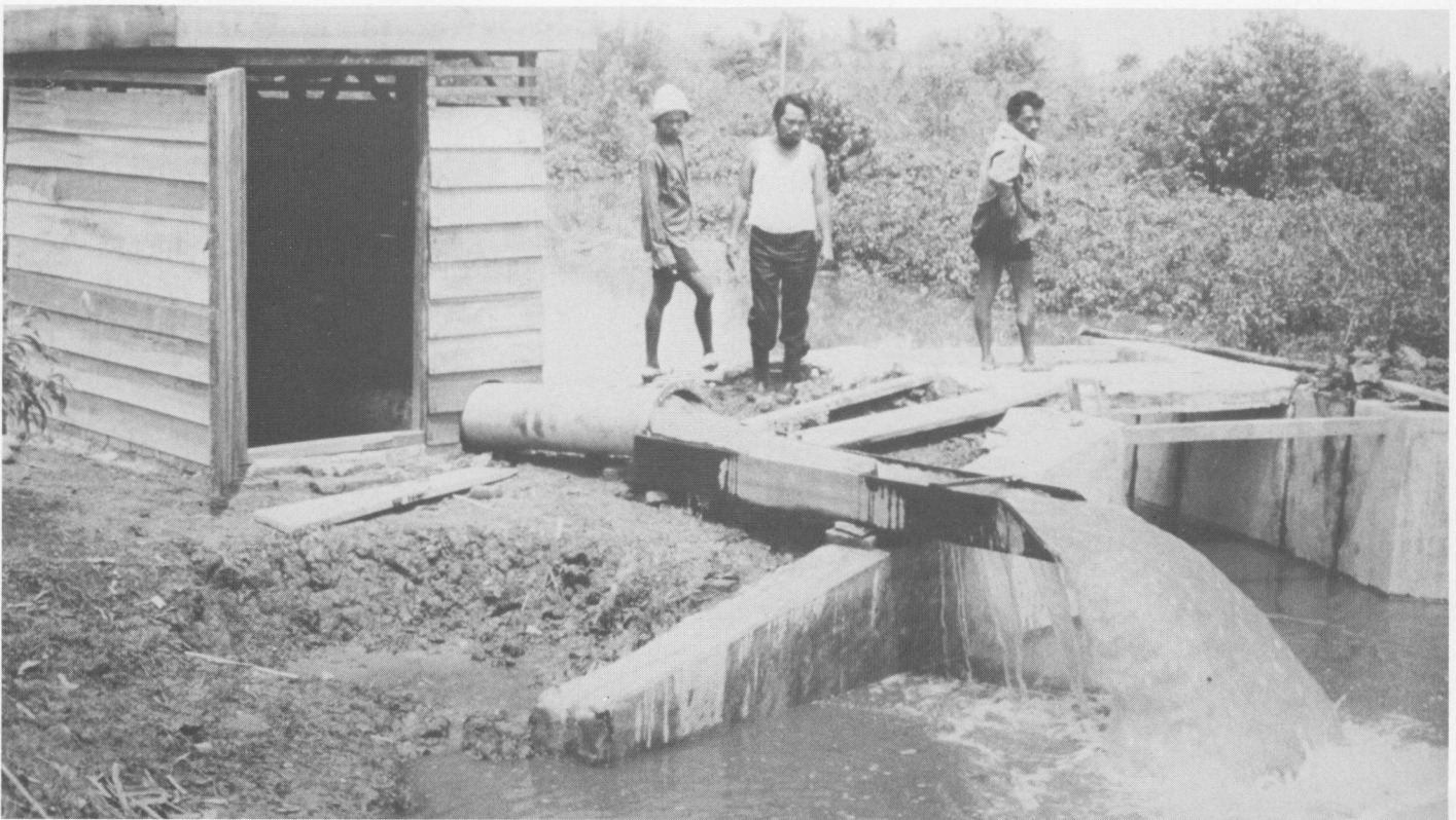
Pumping water from tidal channel to pond supply canal.
