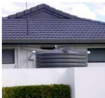
Rainwater tank visible
