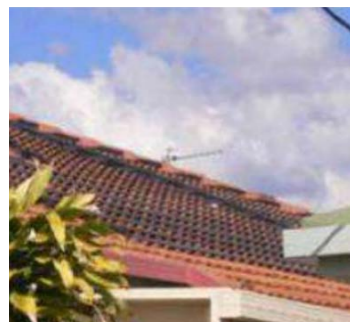
Roof-mounted pool heating visible
