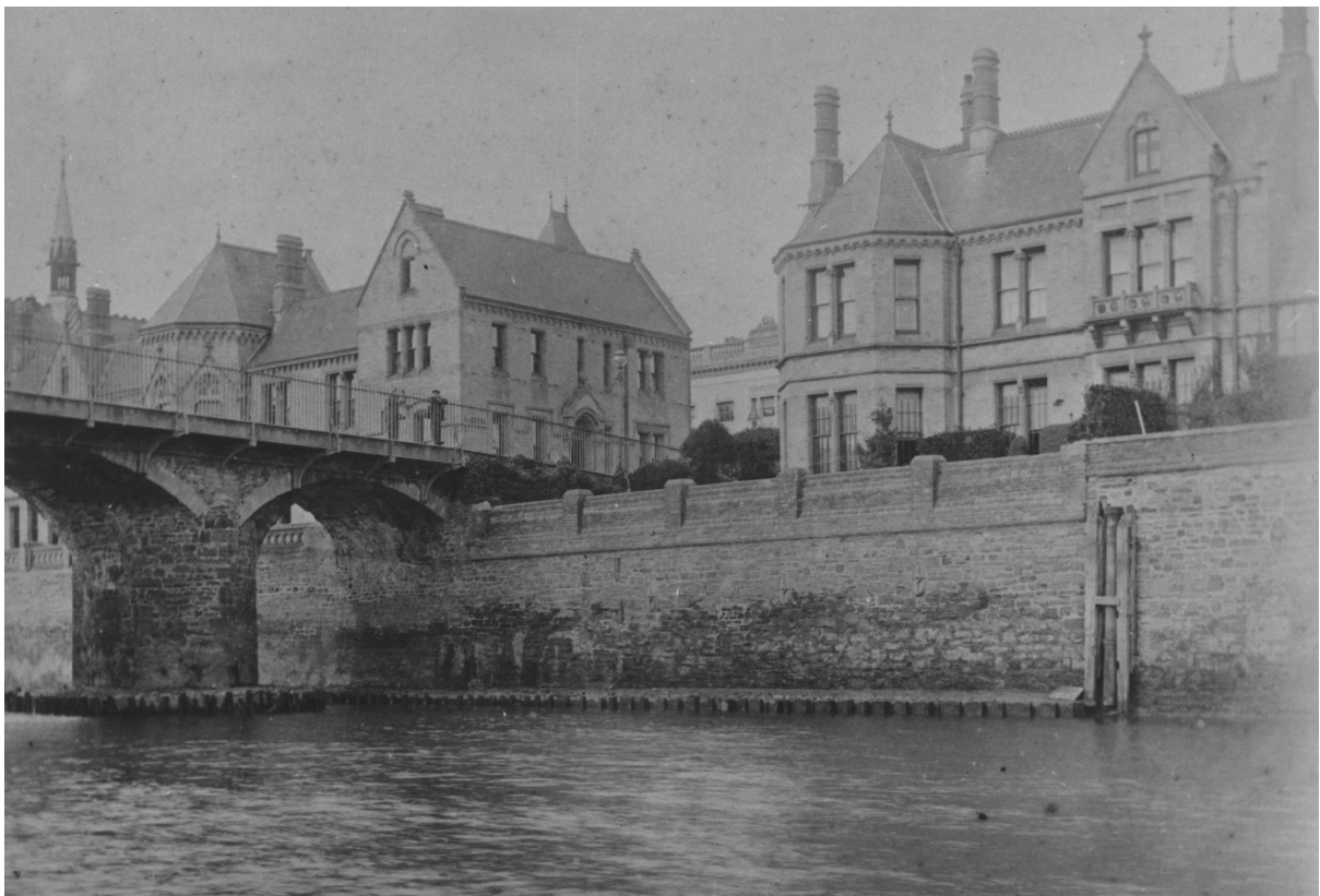
Twon end of the Bridge in 1916 showing the Bridge End Building (demolished in 1963 after sale to the Ministry of Transport)
