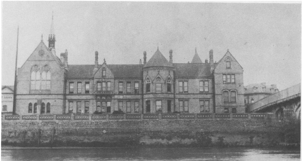
Bridge Chambers – as completed in about 1873. This photograph was taken in 1916
