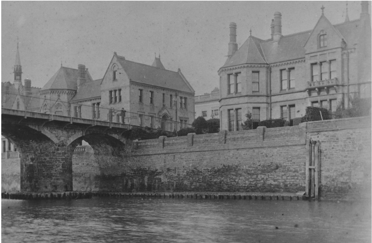
Another 1916 photograph of Bridge End (from the river side), which also give a good view of the piling protection of the river wall and bridge arches.
