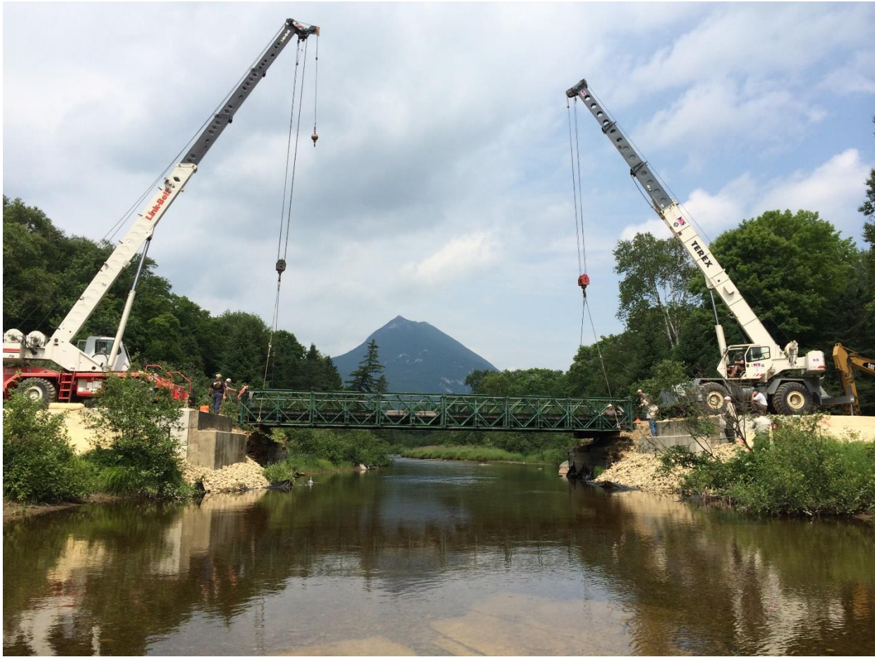
Figure 9 Crews move the Kidney Pond Bridge to new abutments (foreground)
