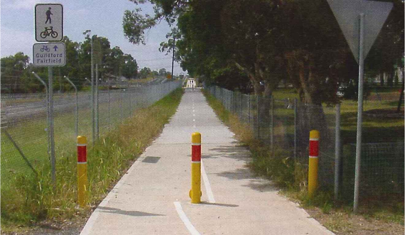
Figure 7.7: Example of a bollard treatment
