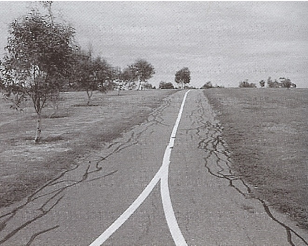
Figure C 2: Asphalt path requiring maintenance
