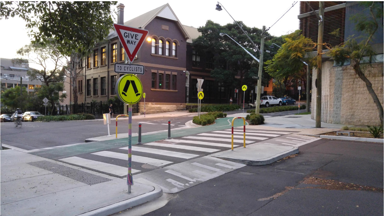
Figure 7.2: Example of an intersection where a separated pedestrian path crossing and a separated bicycle path crossing has priority across a local street
